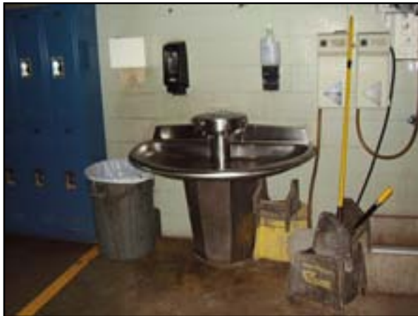
Plumbing: Replace Lavatory Wash Fountains
