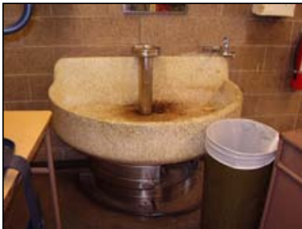
Plumbing: Replace Lavatory Wash Fountains and Column Showers
