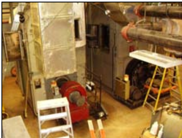
HVAC: Boiler Room Upgrades
