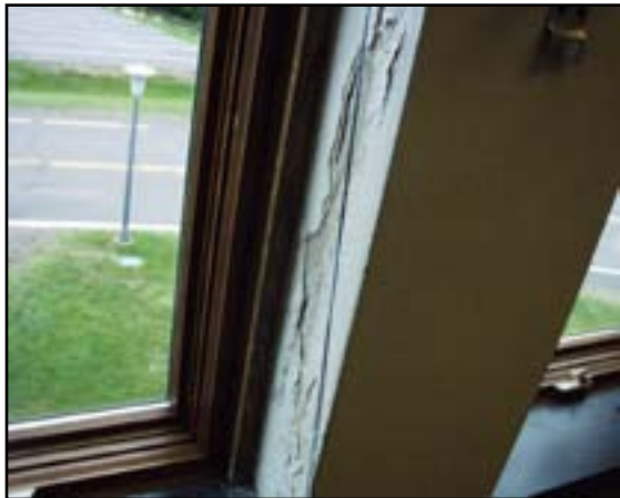
Superstructure: Repair Damaged Plaster
