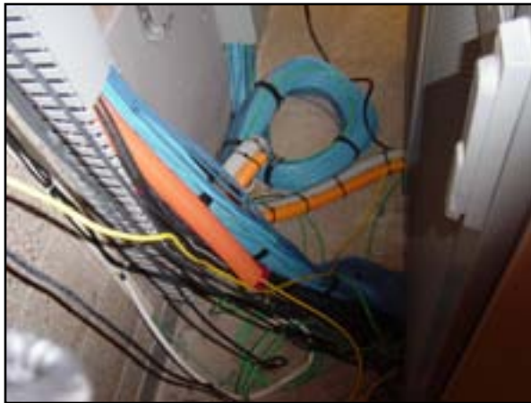
Communication and Security: Cabling Upgrade
