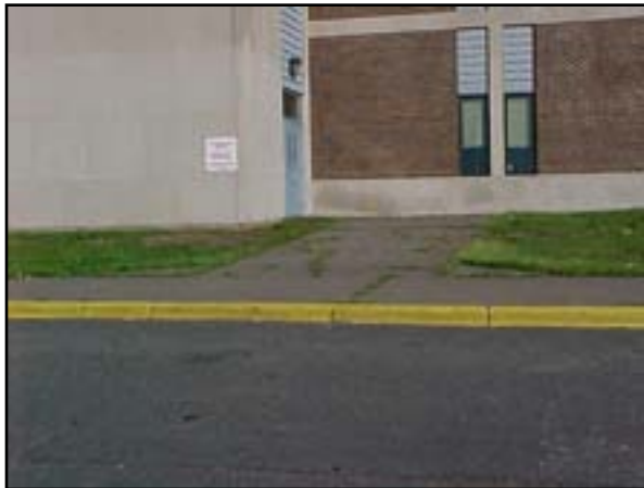
Site Improvements: Accessibility
