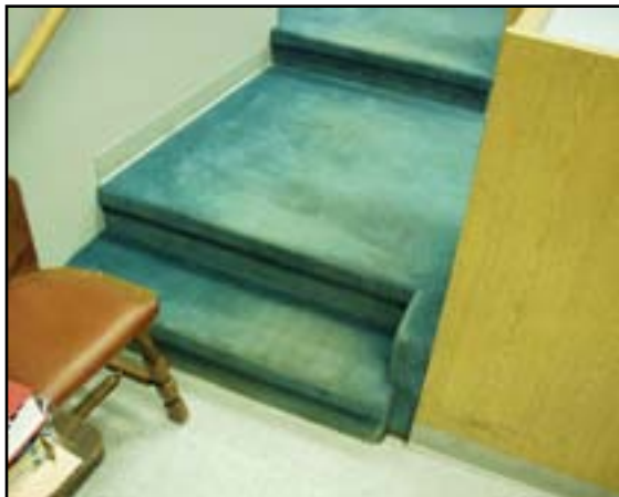
Floor Finishes: Replace Carpet
