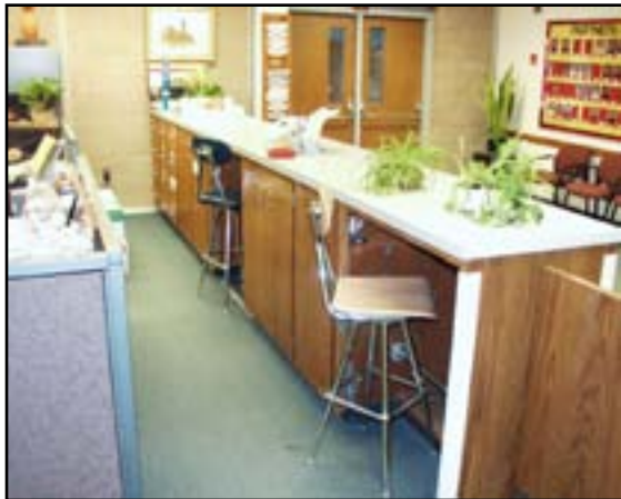
Equipment and Furnishings: Replace Office Main Counter
