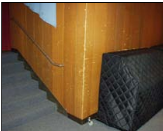
Wall Finishes: Refinish Wood Wall in Auditorium
