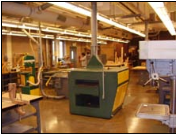
HVAC - Upgrade Dust Collector Filtration
