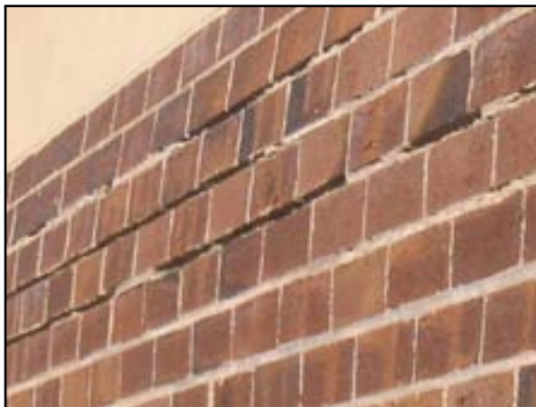
Exterior Walls: Roof-Level Wall Restoration
