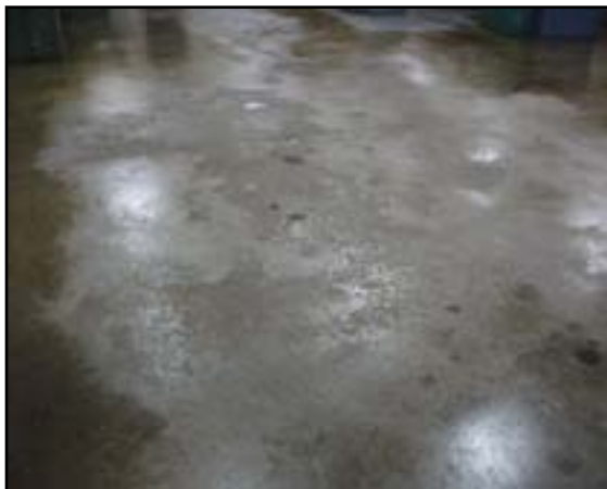
Floor Finishes: Repair Deteriorated Concrete
