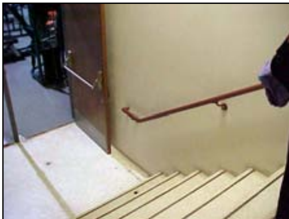
Interior Construction: Accessibility
