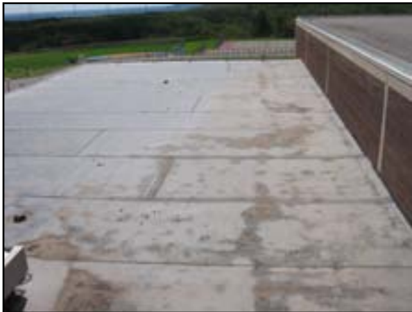
Roof System: Replace Roof
