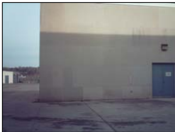
Emergency Power Distribution: Generator Backup
