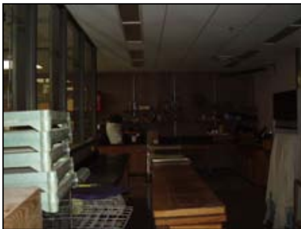
HVAC: Upgrade Ventilation for the Classroom and Admin Areas
