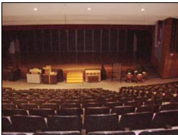
Stairs: Add Handrails
