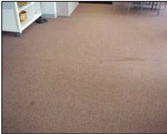
Floor Finishes: Replace Carpet
