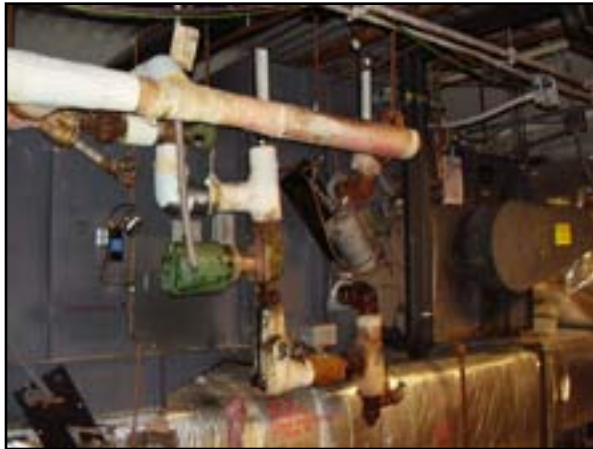
HVAC: Add Propylene Glycol to Heating System
