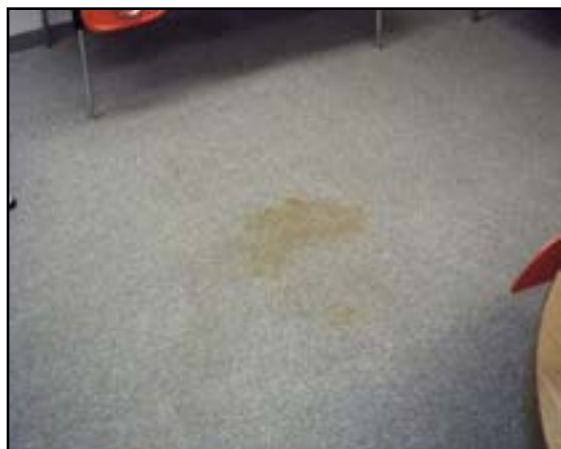
Floor Finishes: Replace Carpet
