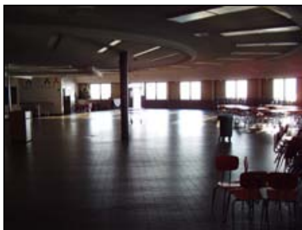
HVAC: Upgrade Ventilation for the Cafeteria and Lower Level Social Studies/Child Care Areas
