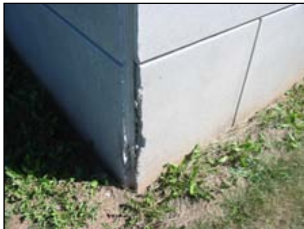
Exterior Walls: Wall Restoration
