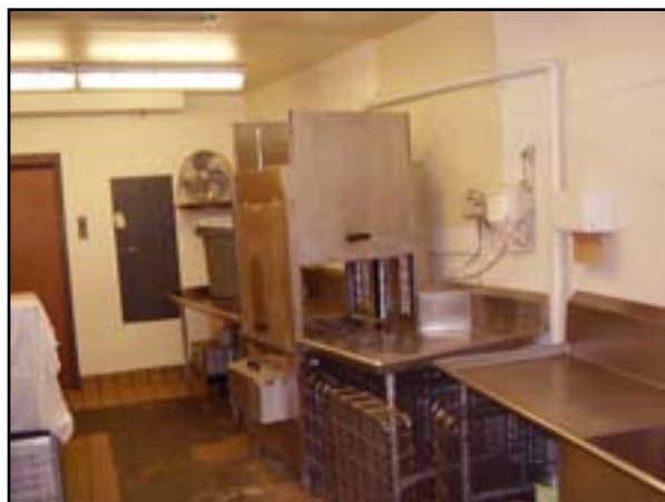
HVAC: Add Exhaust Hood to Dishwasher
