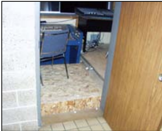
Superstructure: Refurbish Auditorium Projection Booth (Control Room)
