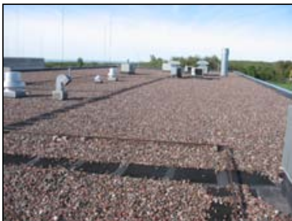
Roof System: Replace Roof
