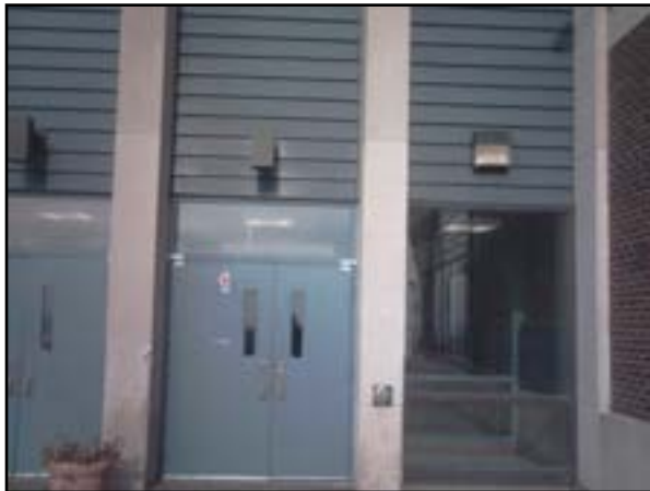
Communication and Security: Access Control
