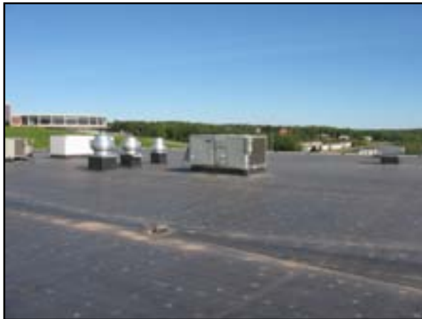
Roof System: Replace Roof
