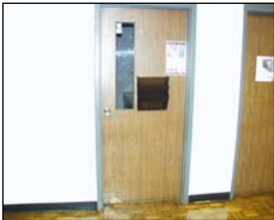
Interior Doors: Replace All Plastic Laminate Interior Doors and Hardware
