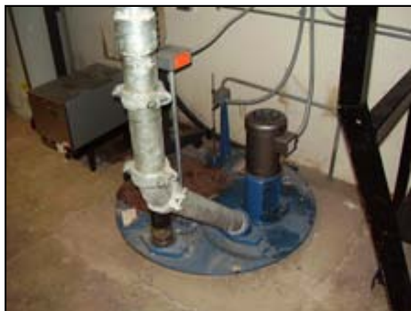
Plumbing - Sump Pump Replacement
