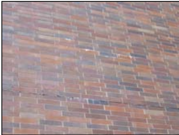
Exterior Walls: Wall Restoratiion -
