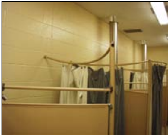
Fittings: Replace Shower Curtain Frames/ Curtains
