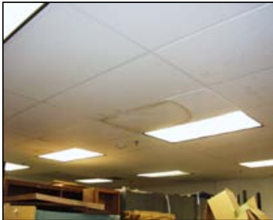
Ceiling Finishes: Replace Suspended Ceiling Tile
