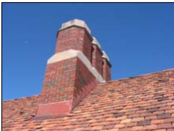
Exterior Walls: Chimney Restoration
