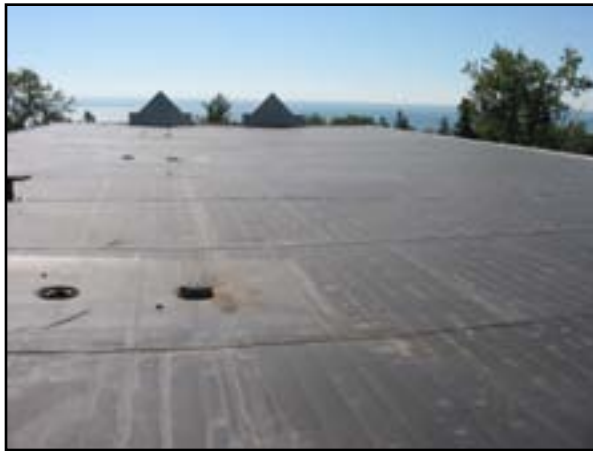
Roof System: Replace Roof
