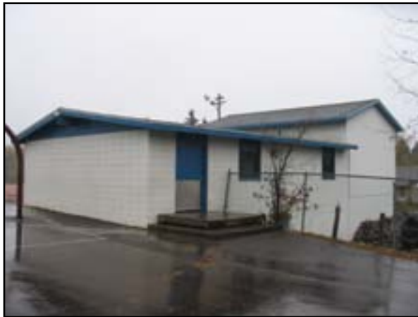
Exterior Walls: Wall Restoration
