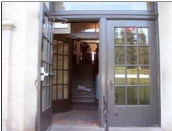
Exterior Doors: Replace Existing Entry Doors
