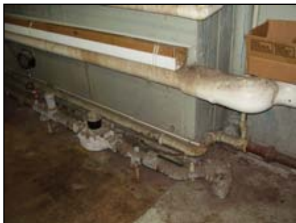
Plumbing: Replace galvanized domestic water piping
