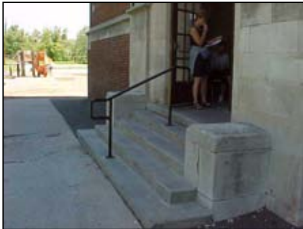
Site Improvements: Accessibility
