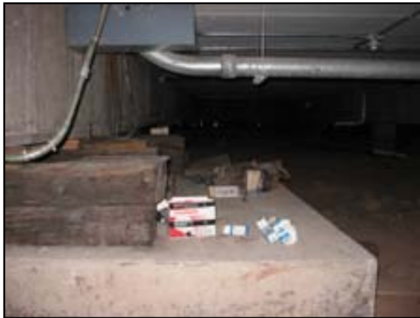
Service Tunnels: Floor Vapor Barrier
