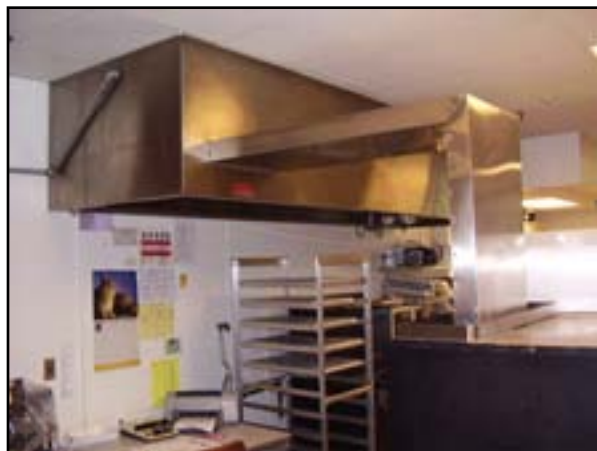
HVAC: Replace Kitchen Grease Exhaust Hoods
