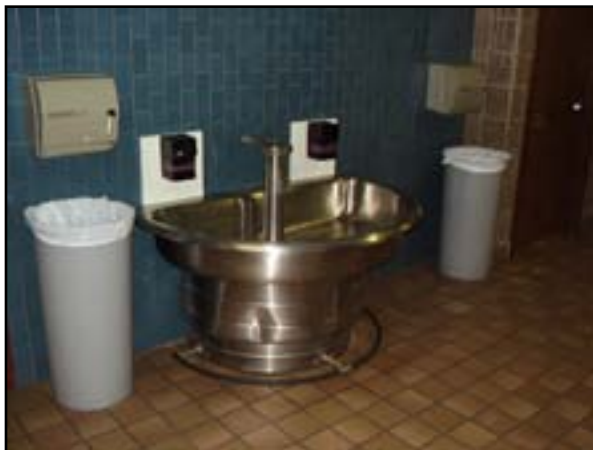
Plumbing: Replace Lavatory Wash Fountains
