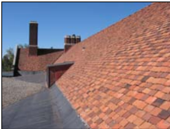
Roof System:Replace Roof
