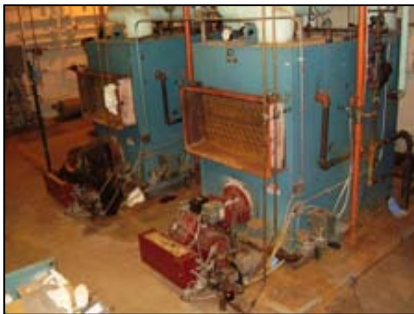
HVAC: Heating System Conversion - Steam to Hot Water
