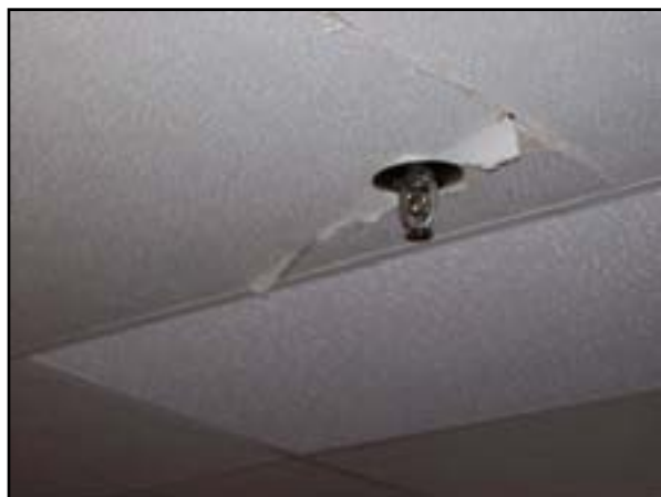
Ceiling Finishes: Replace 2x4 Ceiling Panels
