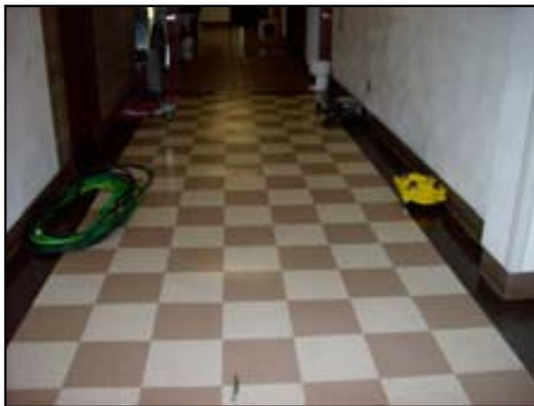
Floor Finishes: Replace Linoleum Tile
