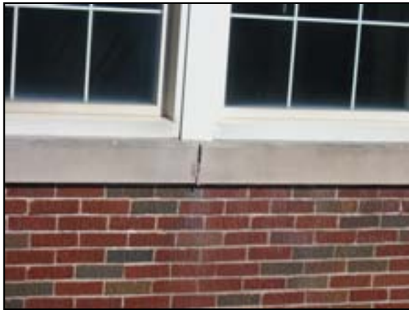
Exterior Walls:Wall Restoration
