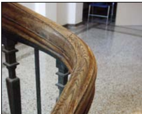
Wall Finishes: Refinish Stair Handrails
