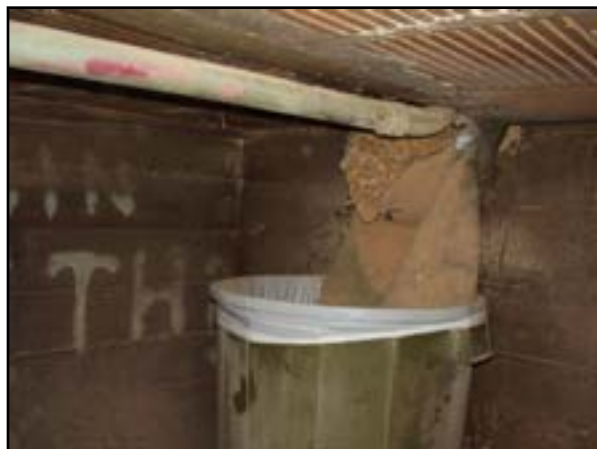
HVAC - Upgrade Ventilation and Replace Wood Shop Dust Collector and Upgrade Weld Hood Exhaust
