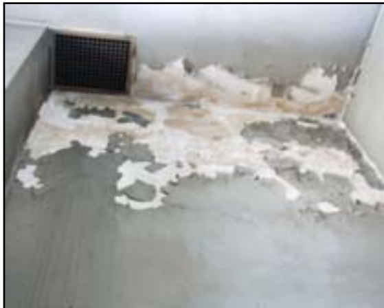
Wall Finishes: Miscellaneous Plaster Repairs
