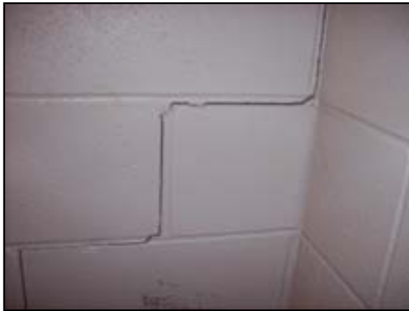
Exterior Walls: Repair Cracks in Masonry Walls
