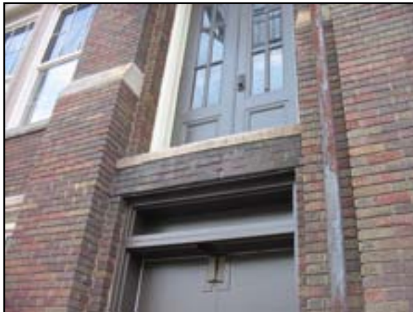
Exterior Walls: Grade-Level Wall Restoration
