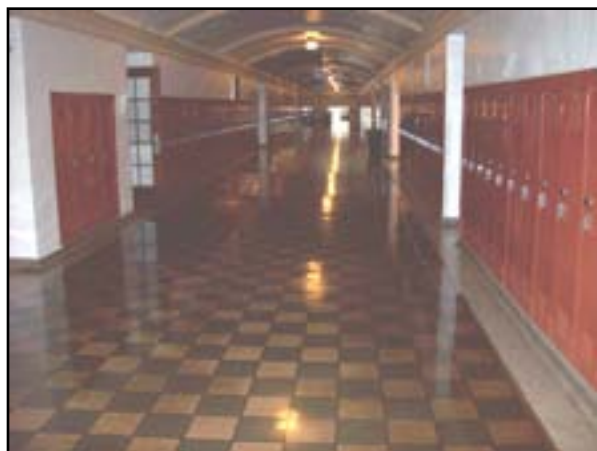
Floor Finishing: Replace Corridor Floor Tile
