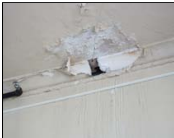
Wall Finishes: Miscellaneous Plaster Repairs
