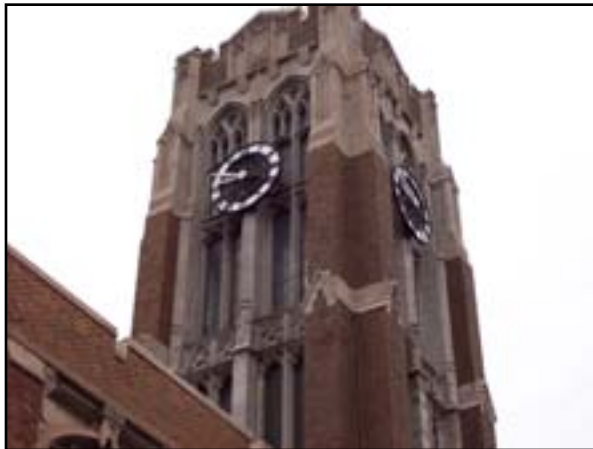
Exterior Windows: Replace Clock Tower Windows
