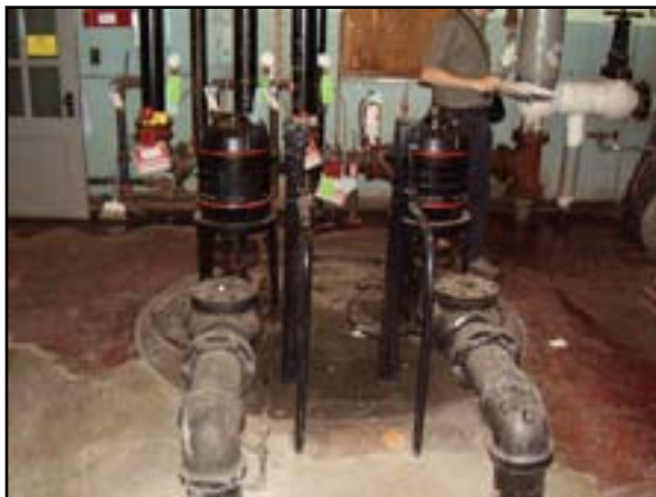
Plumbing - Sump Pump Replacement
