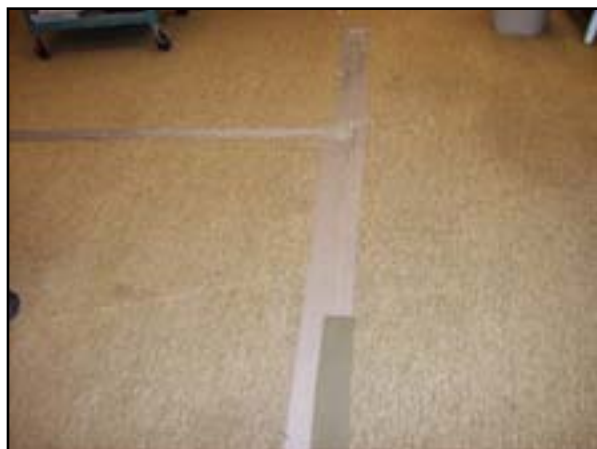
Floor Finishes: Replace Carpet
