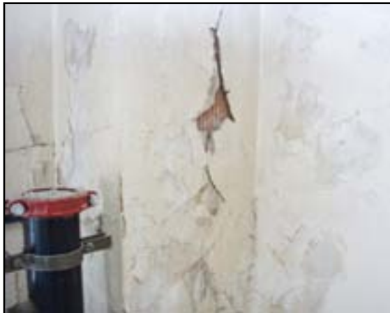
Wall Finishes: Miscellaneous Plaster Repairs
