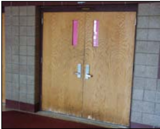
Interior Doors: Replace Wood Doors
