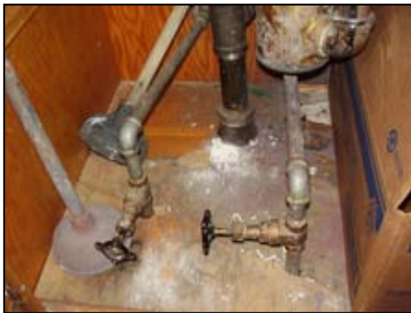
Plumbing: Replace Galvanized Domestic Water Piping
