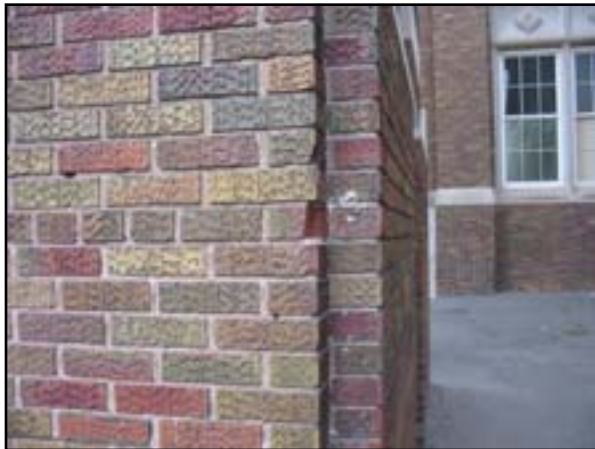
Exterior Walls: Wall Restoration
