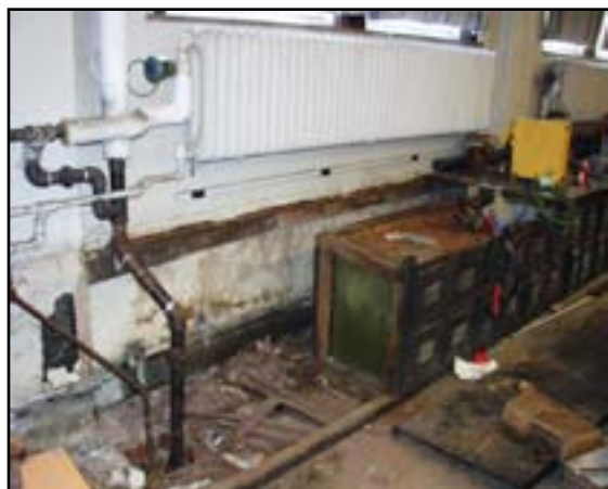
Equipment and Furnishings: Replace Countertops and Project Lockers
