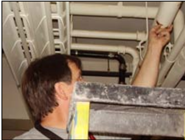
Plumbing: Replace Sanitary Sewer Mains serving the Science Areas
