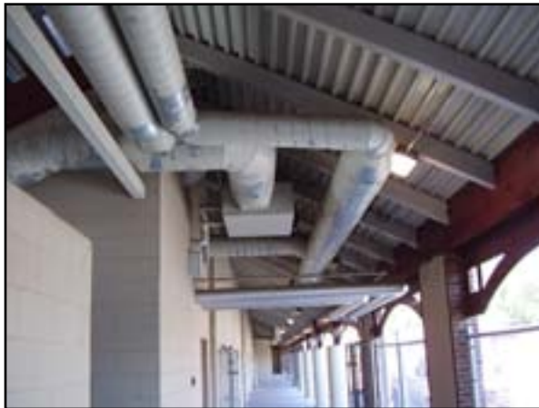
Ceiling Finishes: Paint Surfaces
