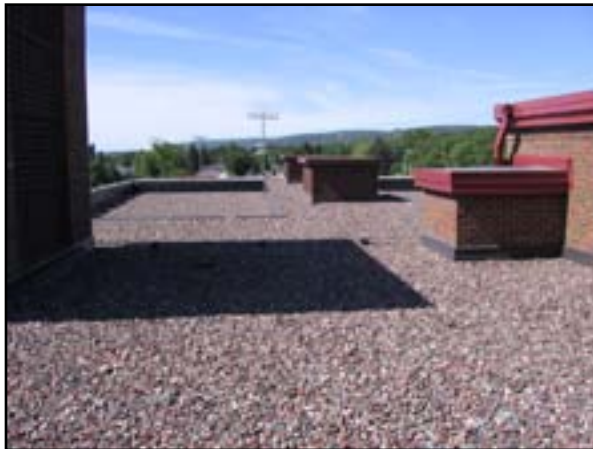
Roof System: Replace Roof
