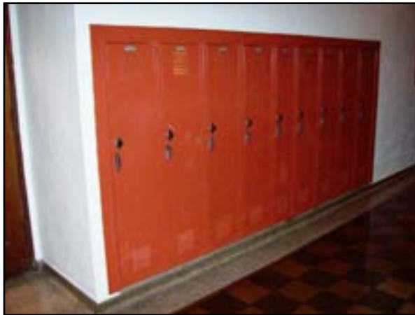
E-Equipment and Furnishings: Replace Lockers -
