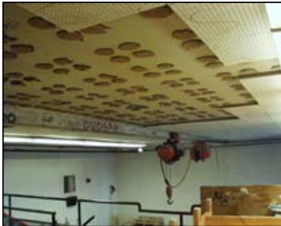
Superstructure: Renovate Ceramics Classroom
