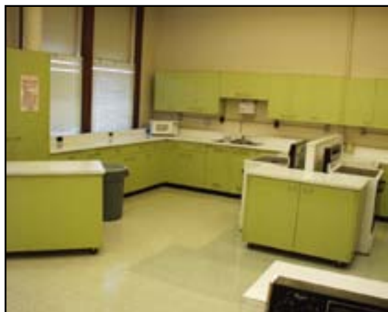
Equipment and Furnishings: Refurbish Cabinets and Countertops
