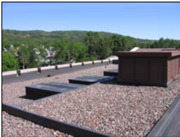
Roof System: Replace Roof
