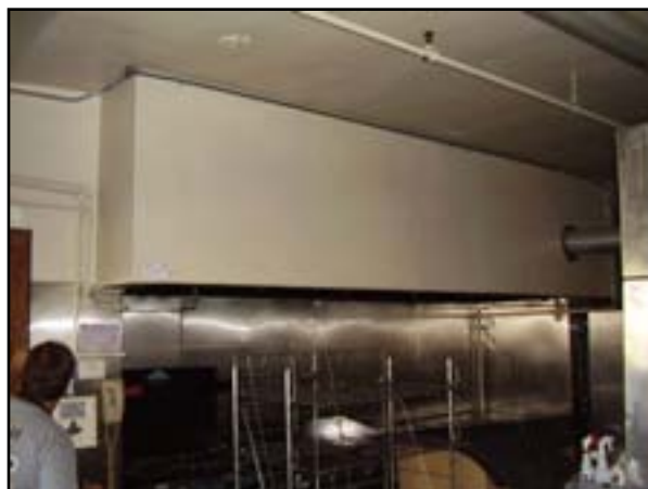
HVAC: Replace Kitchen Grease Exhaust Hood / Add Kitchen Make Up Air
