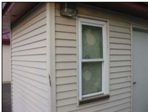
Exterior Walls: Grade-Level Restoration
