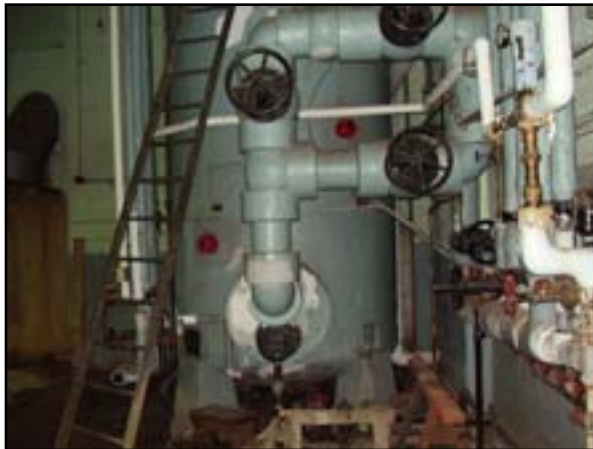
Plumbing: Replace Domestic Water Heat Exchanger for Domestic Hot Water
