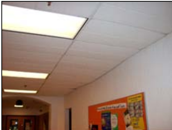
Ceiling Finishes: Replace 2x4 Acoustical Tile
