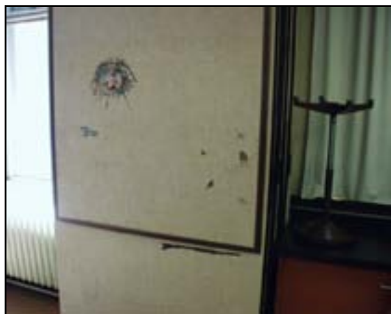
Equipment and Furnishings: Replace Folding Partition
