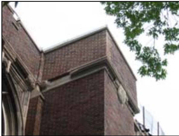
Exterior Walls: Grade-Level Wall Restoration -
