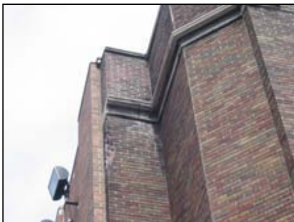
Exterior Walls: Wall Restoration
