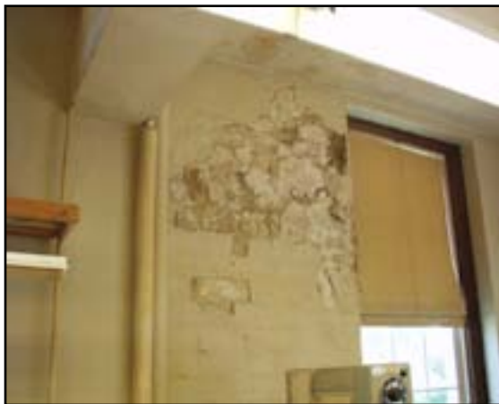
Wall Finishes: Repair Damaged Plaster
