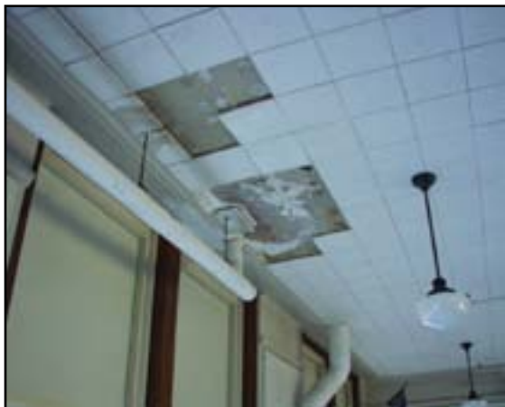
Ceiling Finishes: Replace Ceiling in Cafeteria
