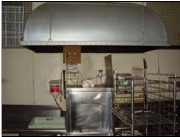
HVAC: Replace Dishwasher Exhaust Hood
