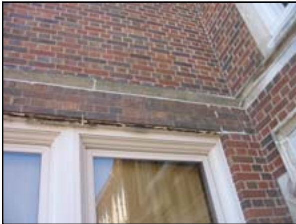
Exterior Walls: Grade-Level Wall Restoration -
