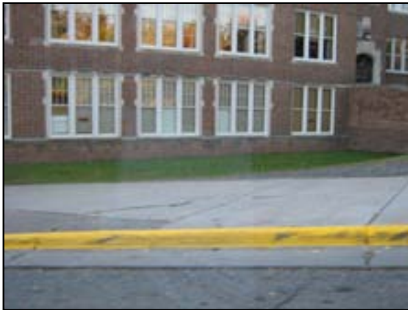
Front Entrance Sidewalk
