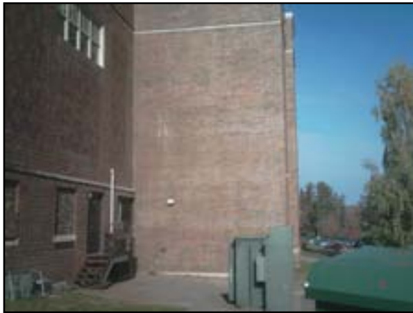
Emergency Power Distribution: Generator Backup
