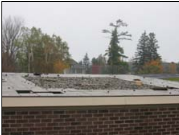
Roof System: Replace Roof
