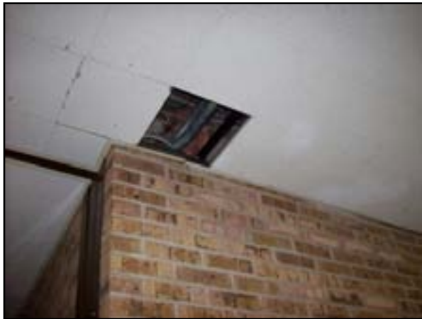
Ceiling Finishes: Repair Splined Ceiling
