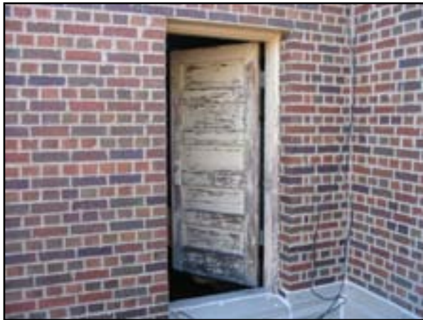
Exterior Walls: Roof-Level Wall Restoration -
