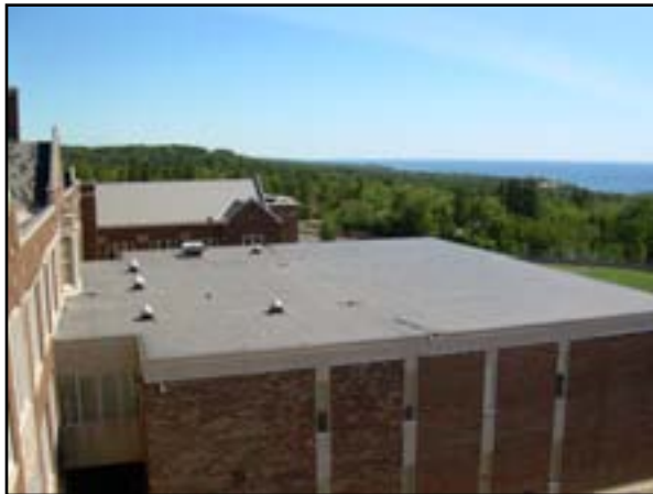
Roof System: Replace Roof
