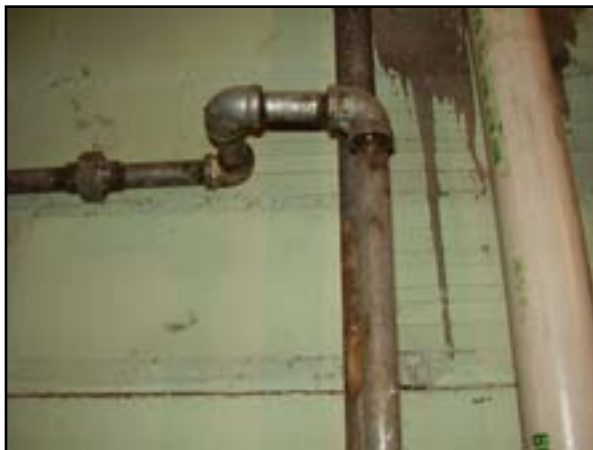
Plumbing: Replace Galvanized Domestic Water Piping
