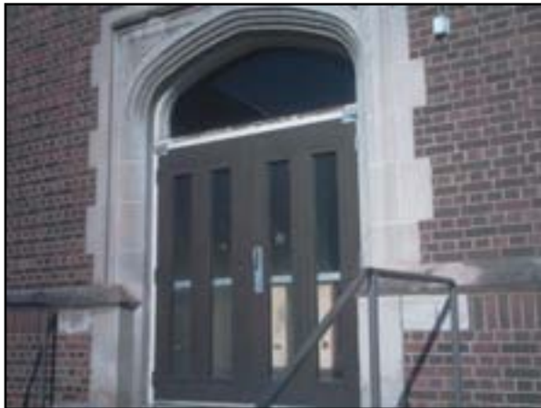
Communication and Security: Access Control
