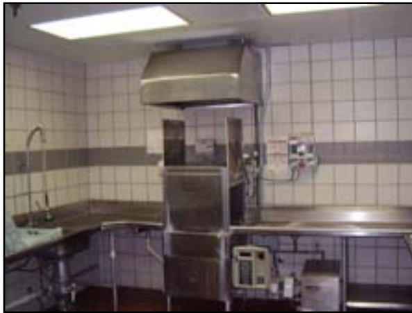
HVAC: Replace Dishwasher Exhaust Hood
