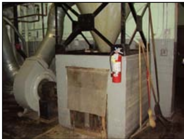
HVAC - Upgrade Ventilation and Replace Wood Shop Dust Collector
