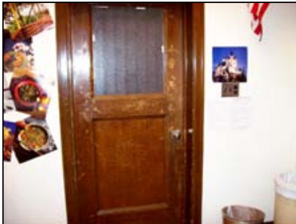
Interior Doors: Replace Wood Doors
