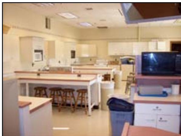
Wall Finishes: Paint Interior
