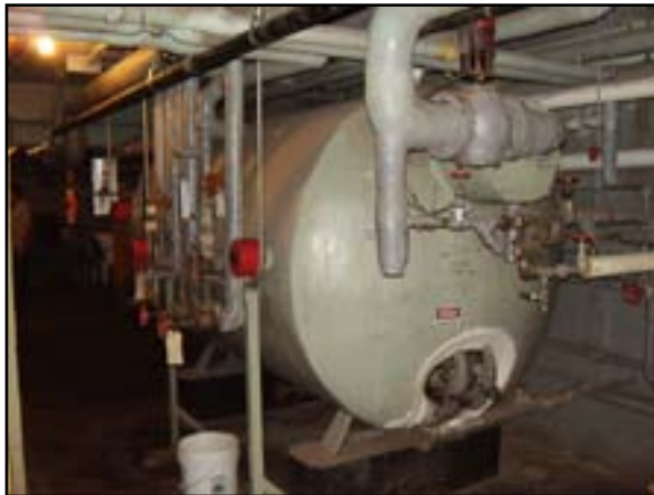
Plumbing: Add Domestic Water Heat Exchanger
