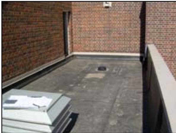
Roof System: Replace Roof
