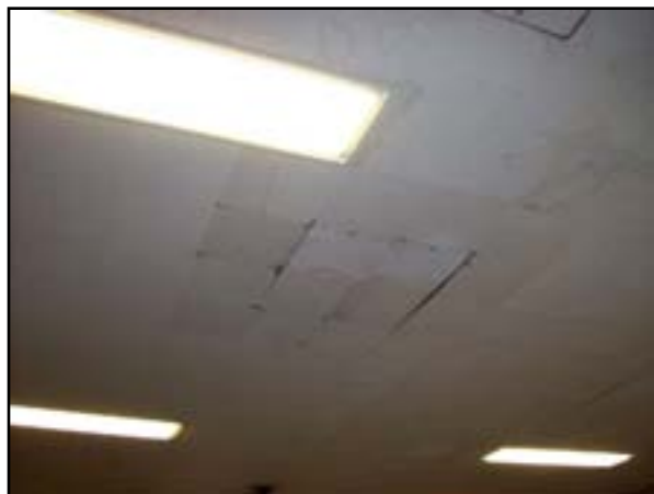
Ceiling Finishes: Replace 12x12 Acoustical Tile
