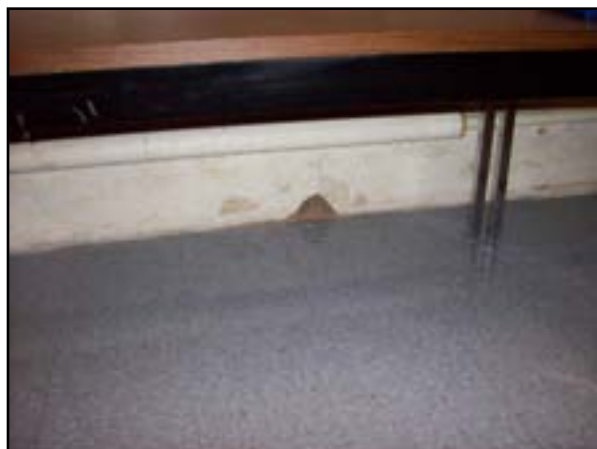
Wall Finishes: Repair Wall Leak
