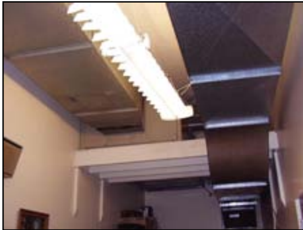
HVAC: Upgrade Office Ventilation and Add Dehumidification
