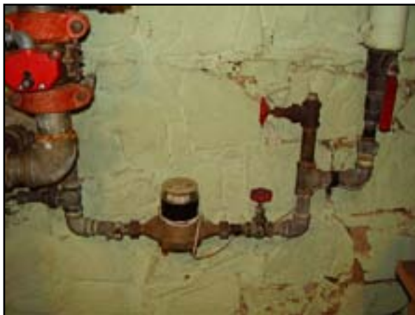
Plumbing: Replace Galvanized Domestic Water Piping
