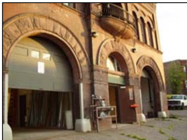
HVAC: Heating System Upgrade - Garages
