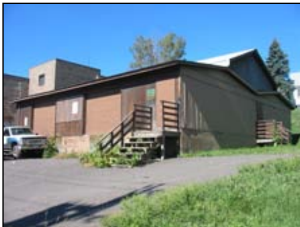
Exterior Walls: Grade-Level Wall Restoration
