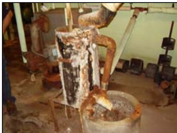
Plumbing - Sand Separator Replacement
