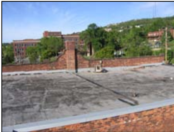
Roof System: Replace Roof
