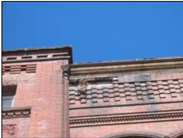
Exterior Walls: Grade-Level Wall Restoration
