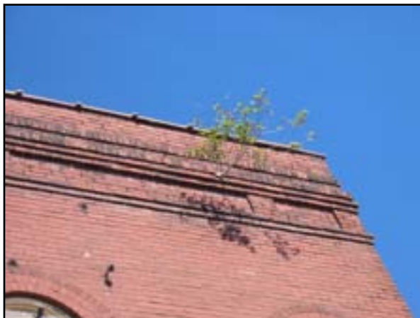
Exterior Walls: Grade-Level Wall Restoration
