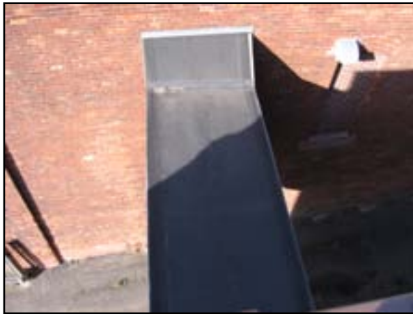
Roof System: Replace Roof
