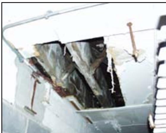
Superstructure: Waterproof Garage 213 Slab
