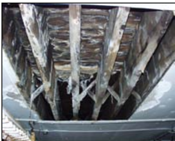
Superstructure: Waterproof Garage 213 Slab
