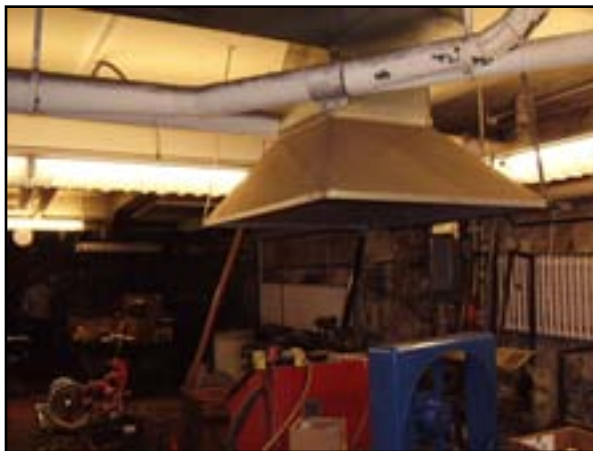
HVAC - Replace Wood Shop Dust Collector and Upgrade Weld Hood Exhaust
