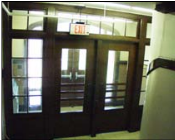
Interior Doors: Replace Vestibule Doors
