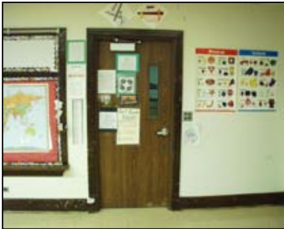
Interior Doors: Replace Classroom Entry Doors
