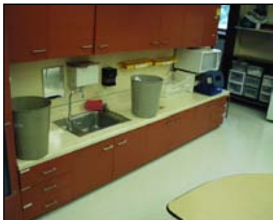
Equipment and Furnishings: Replace Countertops
