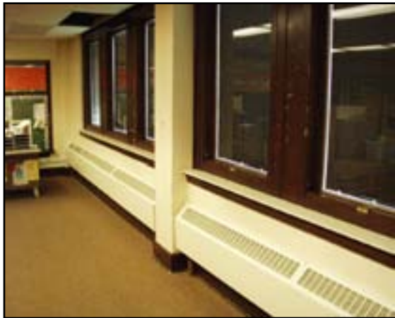
Floor Finishes: Replace All Carpet
