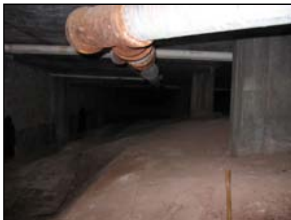
Service Tunnels: Floor Vapor Barrier
