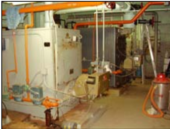
HVAC: Boiler Room Upgrades
