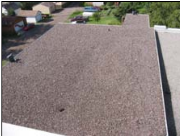
Roof System: Replace Roof
