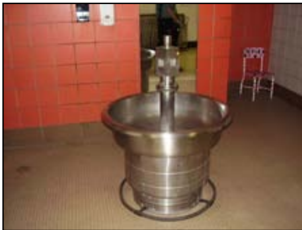
Plumbing: Replace Lavatory Wash Fountains
