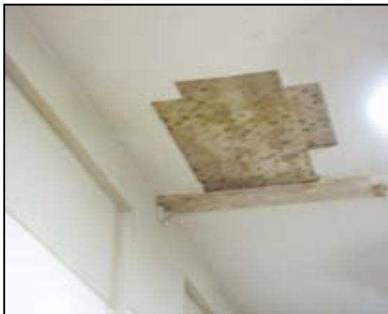
Ceiling Finishes: Replace Gymnasium Ceiling
