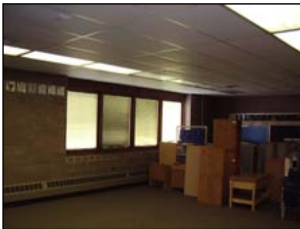
HVAC: Add Dehumidification to the 1991/1993 Additions
