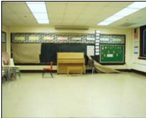
Fittings: Replace Existing Blackboards and Tackboards
