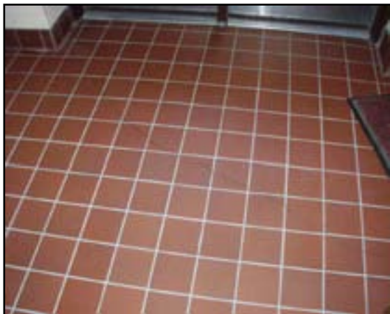
Floor Finishes: Replace Quarry Tile
