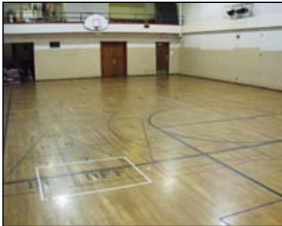
Floor Finishes: Refinish Gymnasium Wood Floor
