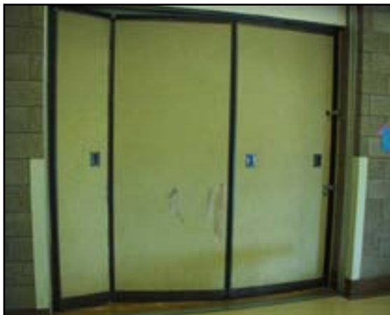
Interior Doors: Replace Folding Doors
