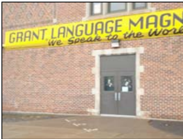
Communication and Security: Access Control
