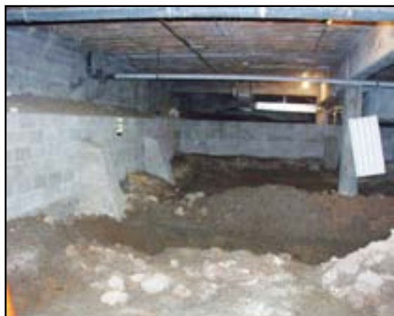
Floor finishes: Install Concrete Slab
