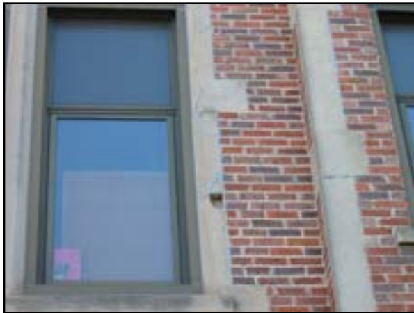
Exterior Walls: Wall Restoration
