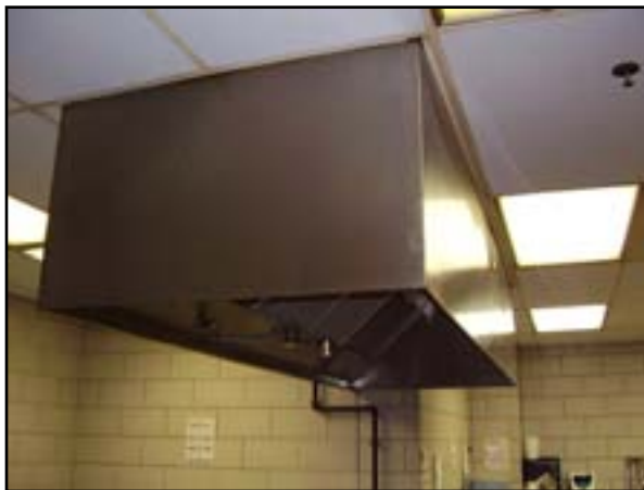
HVAC: Replace Kitchen Grease Exhaust Hood
