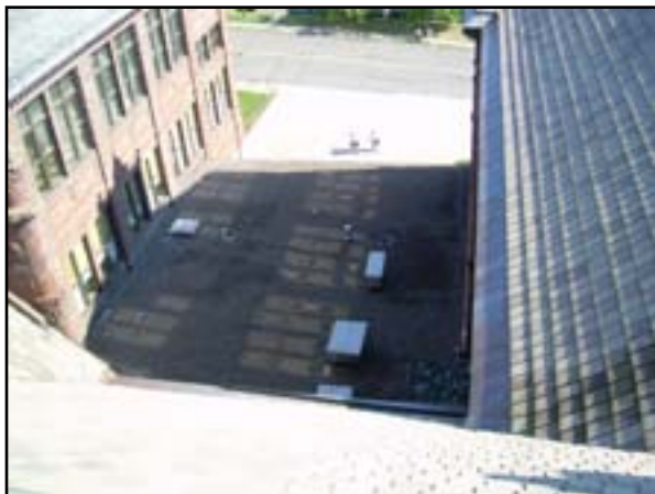
Roof System: Replace Roof
