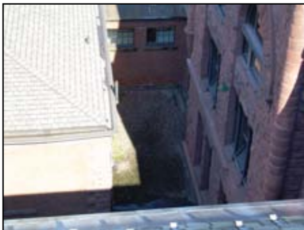
Roof System: Replace Roof
