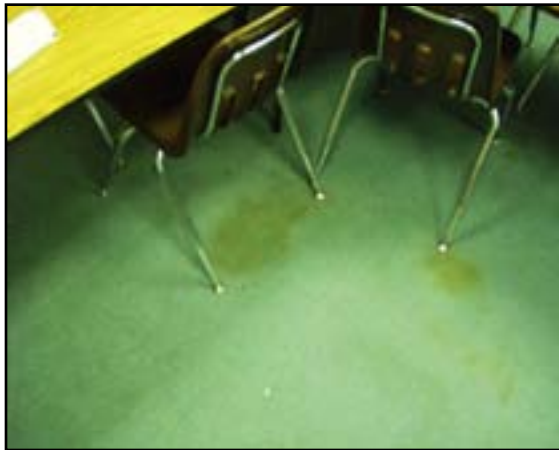
Floor Finishes: Replace Carpet
