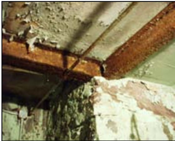
Superstructure: Refinish Steel Beams
