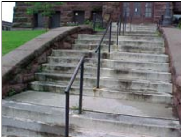
Site Improvements: Accessibility
