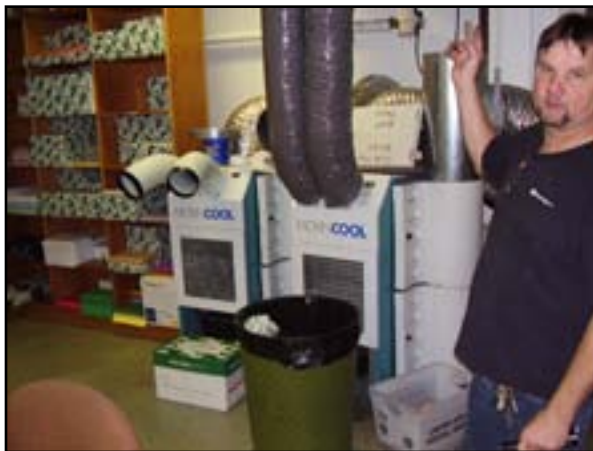
HVAC: Install Ventilation Storage and Print Shop Areas
