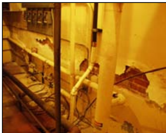
Superstructure: Patch Miscellaneous Walls
