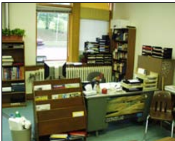
Wall Finishes: Repaint Interior
