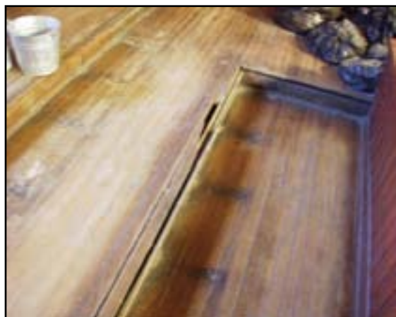
Floor Finishes: Refinish Hardwood Floor
