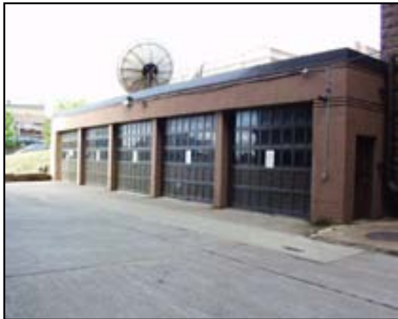
Exterior Doors: Replace Overhead Doors
