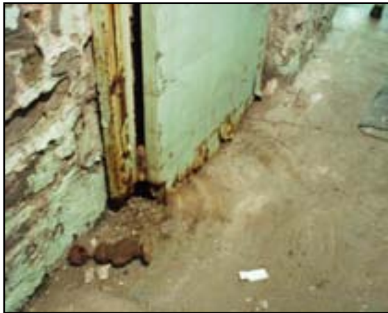
Interior Doors: Replace Boiler Room Door
