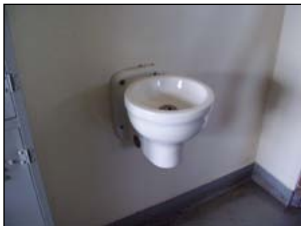
Plumbing: Replace Galvanized Domestic Water Piping
