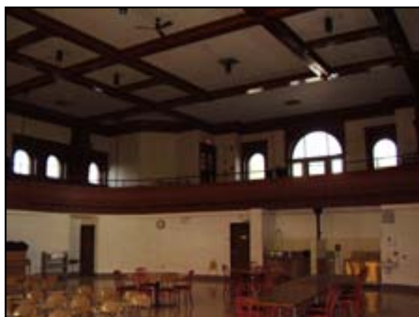
HVAC: Replace Ventilation Venditeria Area
