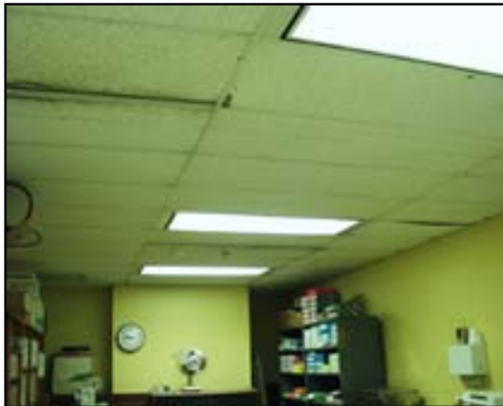
Ceiling Finishes: Replace Suspended Ceiling Tile
