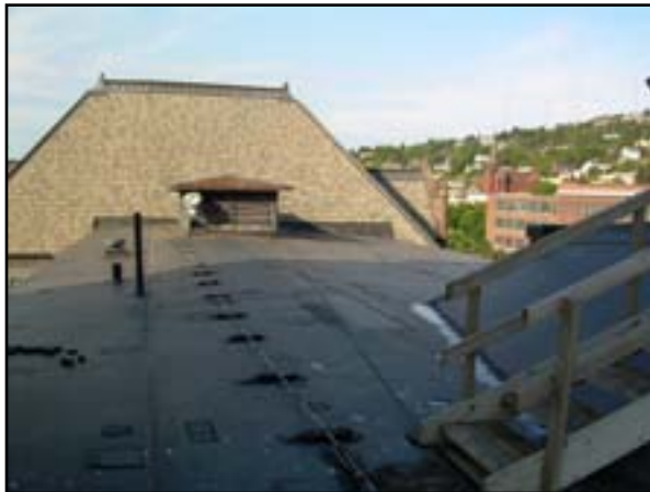
Roof System: Replace Roof
