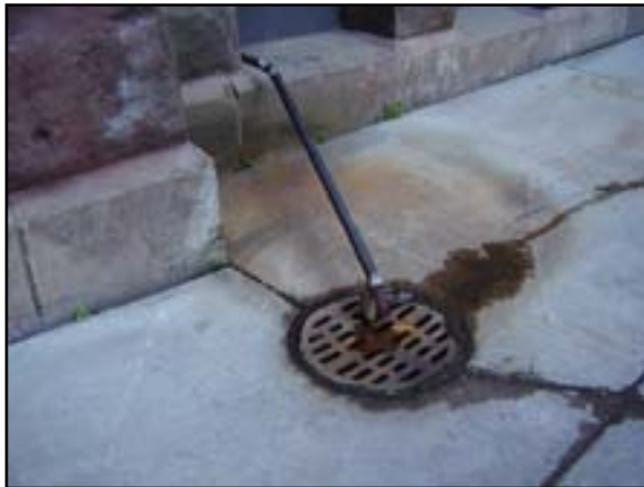
Plumbing - Sump Pump Replacement
