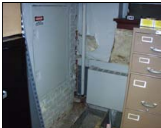
Superstructure: Patch Plaster at Exterior Walls
