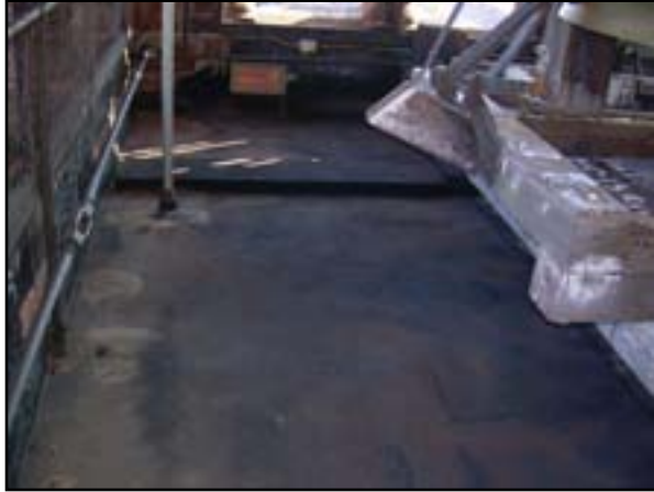
Roof System: Replace Roof
