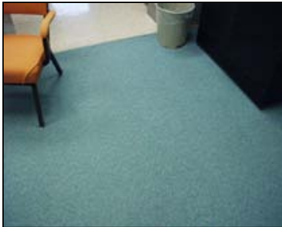
Floor Finishes: Replace Carpet Areas with VCT
