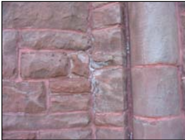
Roof-Level Wall Restoration
