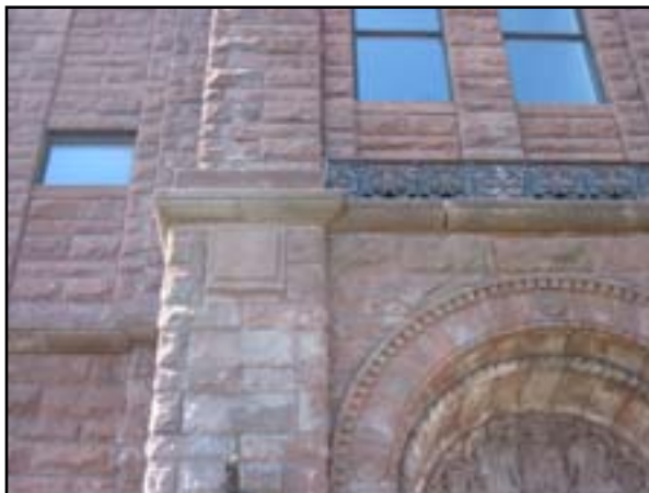
Exterior Grade-Level Walls
