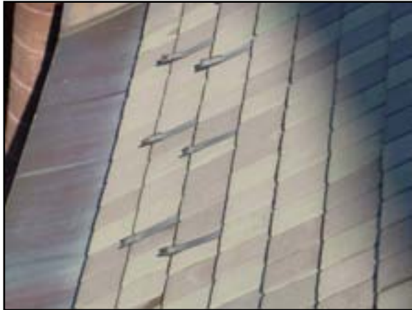
Roof System: Replace Roof
