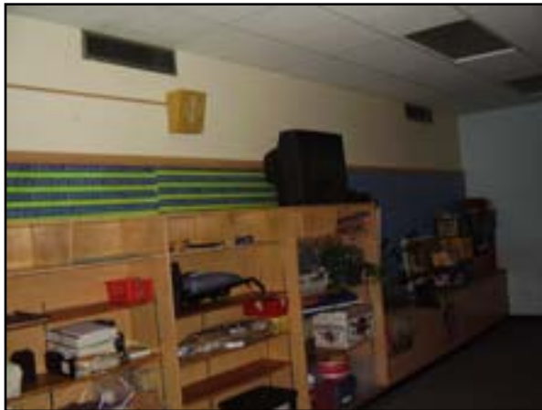
HVAC: Replace Ventilation 1952 Classrooms
