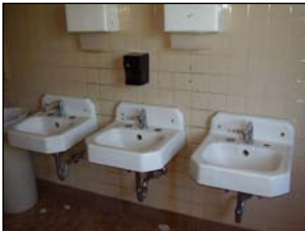
Plumbing: Replace Galvanized Domestic Water Piping
