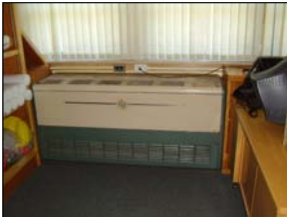
HVAC: Replace Classroom Unit Ventilators
