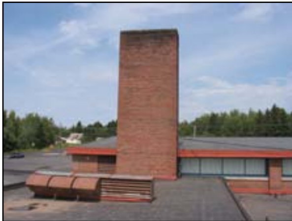
Roof System: Replace Roof
