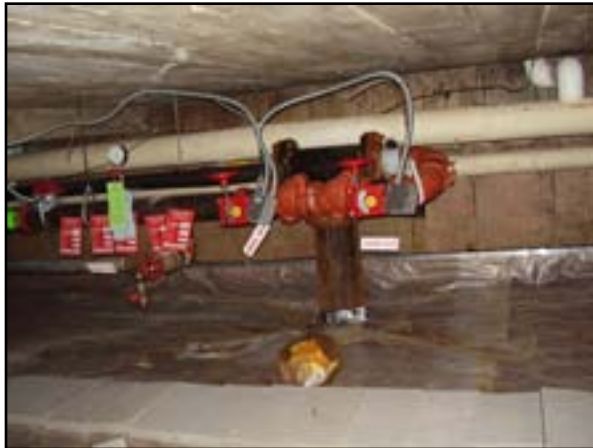
Fire Protection: Provide Improved Sprinkler Service Access
