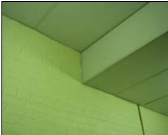
Ceiling Finishes: Replace Acoustical Tile
