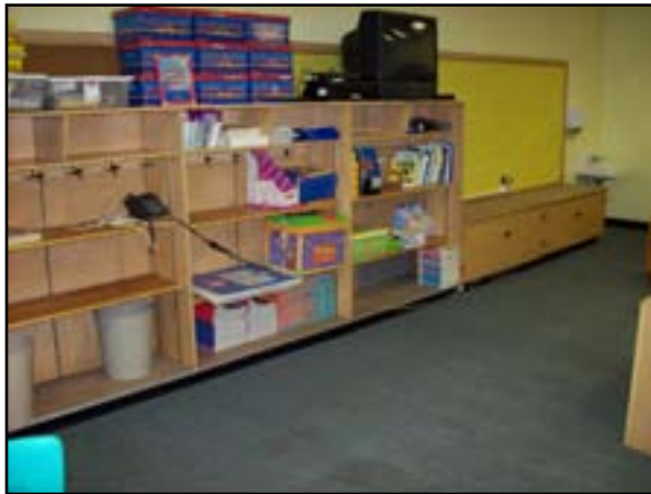
Floor Finishes: Replace Carpet
