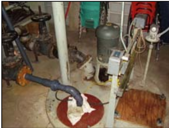
Plumbing - Sewage Ejector Replacement
