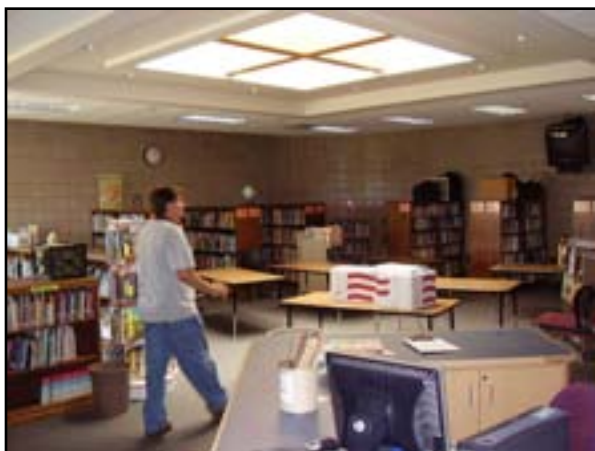
HVAC - 2005 Addition Ventilation Improvements
