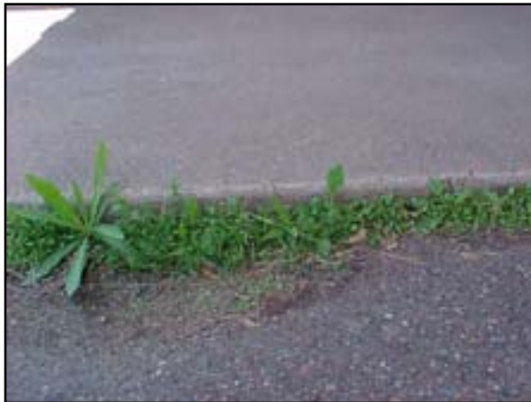
Site Improvements: Accessibility
