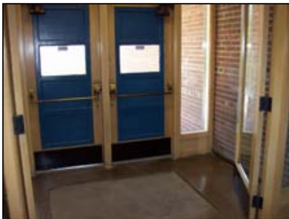
Exterior Doors: Replace Wood Doors
