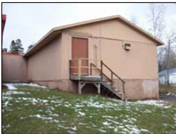
Superstructure: Demolish Relocatable Classroom
