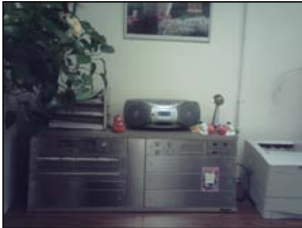
Communication and Security: Public Address and Sound System -
