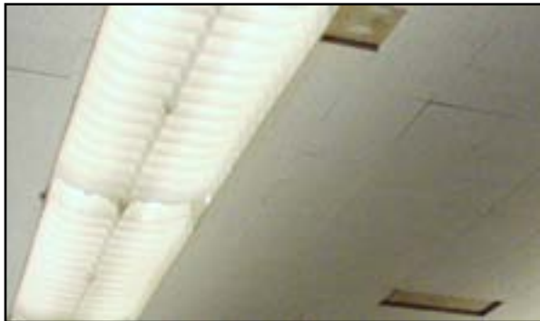
Ceiling Finishes: Replace Acoustical Tile
