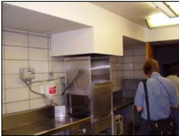
HVAC: Replace Dishwasher Exhaust Hood
