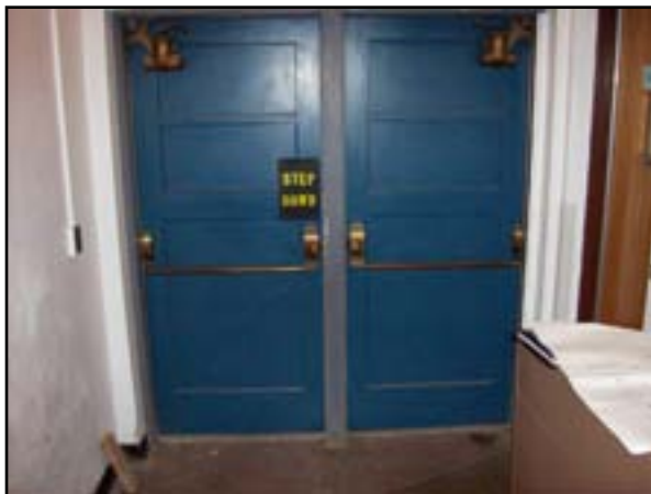
Exterior Doors: Replace Wood Doors
