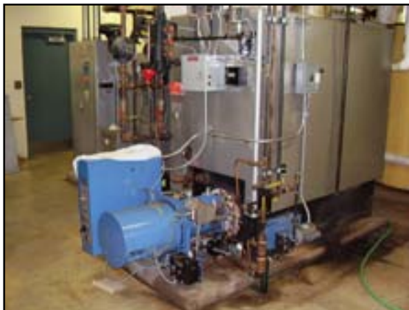
HVAC: Boiler Room Upgrades
