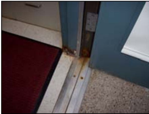
Exterior Doors: Replace Doors and Frames
