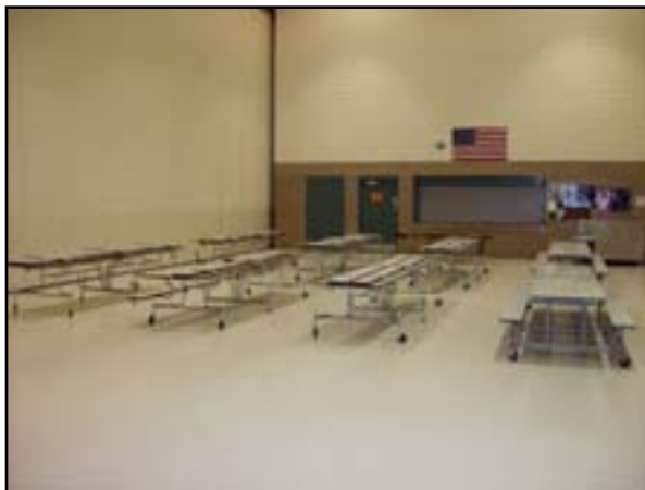
Wall Finishes: Paint Interior Gypsum Board
