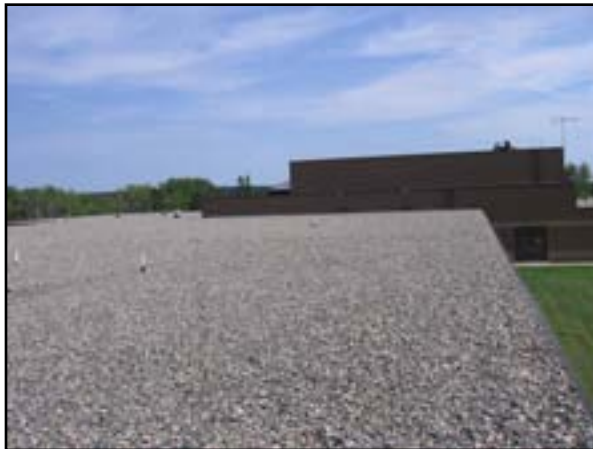
Roof System: Replace Roof
