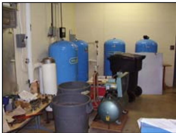
Plumbing: Water Softener Installation
