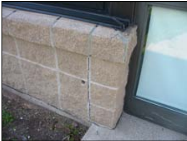
Exterior Walls: Wall Restoration
