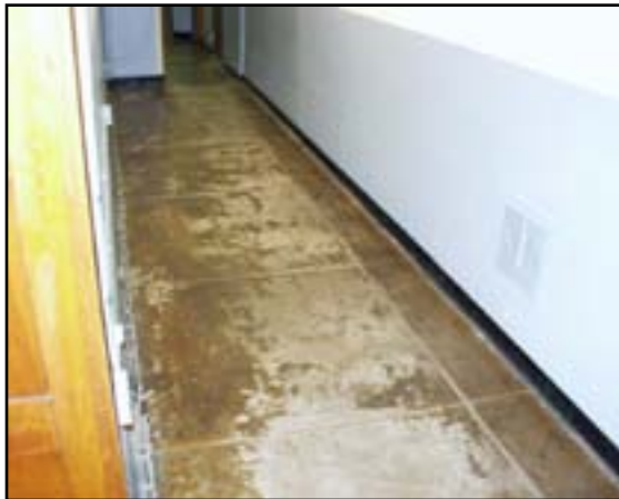
Floor Finishes: Repaint Concrete Floors
