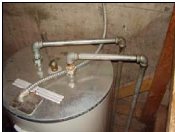
Plumbing: Replace Galvanized Domestic Water Piping
