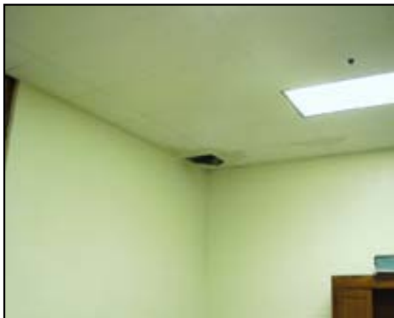
Ceig Finishes: Install New Suspended Acoustical Board Ceiling
