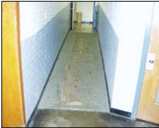
Floor Finishes: Refurbish Lower Level Ramps
