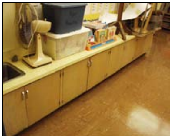
Floor Finishes: Replace Vinyl Asbestos Tile in Classrooms
