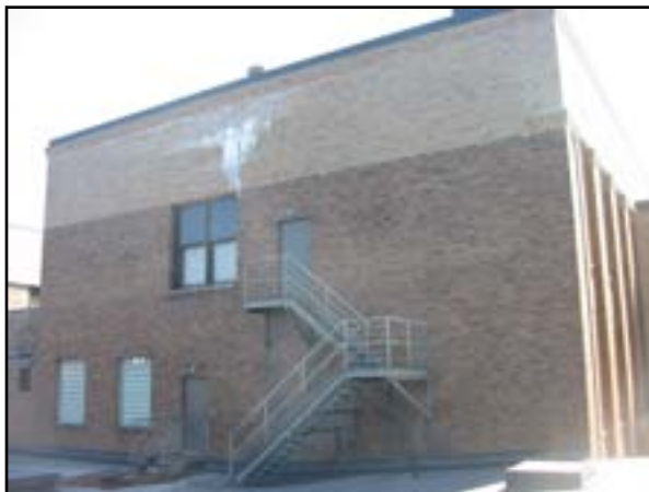
Exterior Walls: Wall Restoration
