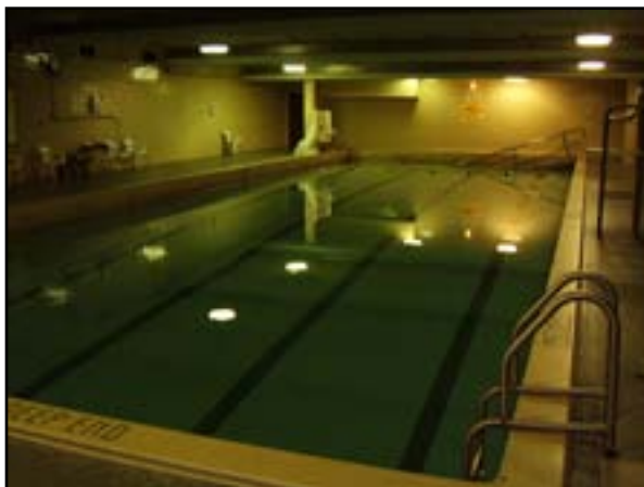
HVAC: Pool Unit Replacement along with an Automatic Pool Cover
