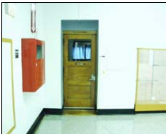
Interior Doors: Replace Classroom Doors 1914 Building
