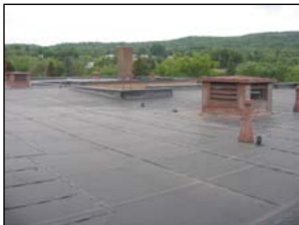
Roof System: Replace Roof
