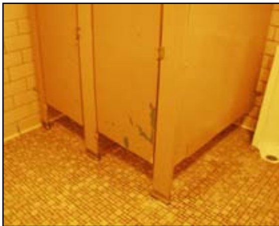
Fittings: Replace Toilet Partitions 11 Locations
