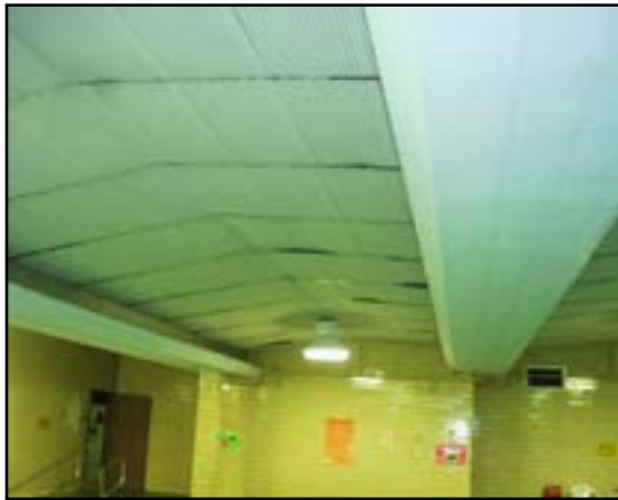
Ceiling Finishes: Replace Ceiling Above Pool
