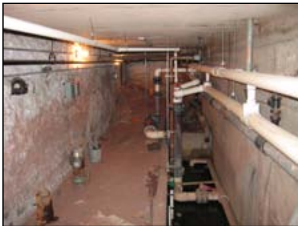
Service Tunnels: Floor Vapor Barrier
