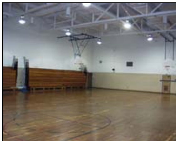
Floor Finishes: Refinish Gymnasium Floor
