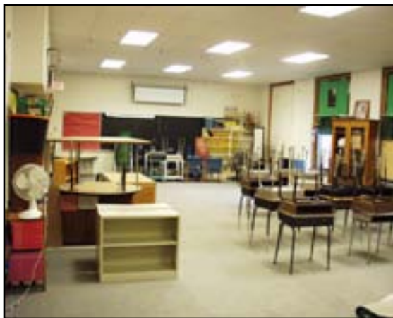
Wall Finishes: Paint Interior
