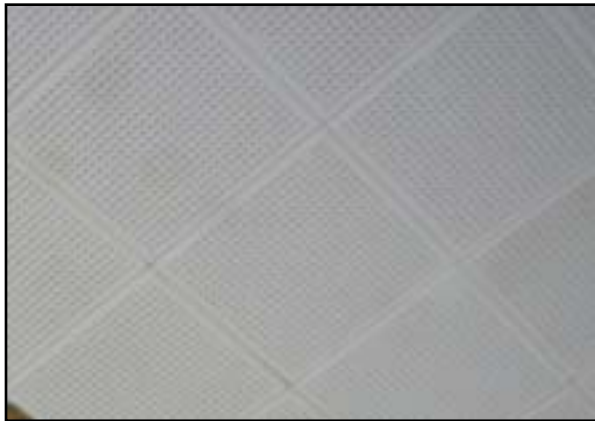
Ceiling Finishes: Replace Cafeteria Ceilings
