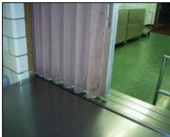
Interior Doors Replace Folding Partition Between Kitchen Cafeteria
