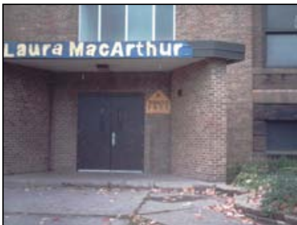
Communication and Security: Access Control
