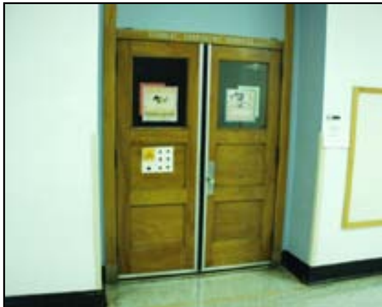
Interior Doors: Replace Hardware and Refinish Doors
