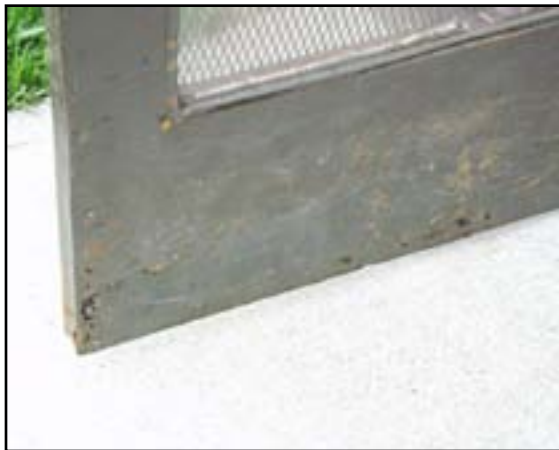
Exterior Doors: Replace Select Hollow Metal Doors
