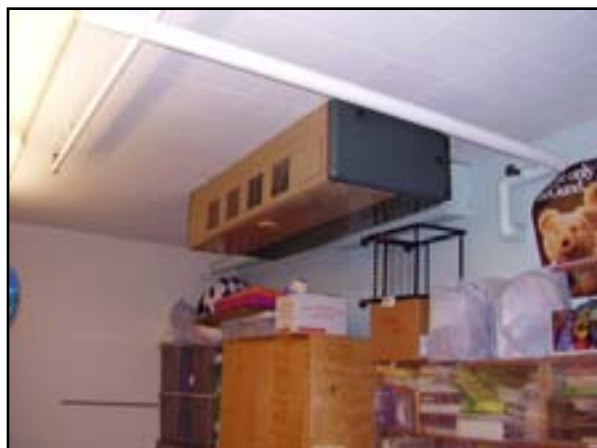
HVAC: Replace Classroom Unit Ventilators
