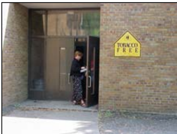
Site Improvements: Accessibility
