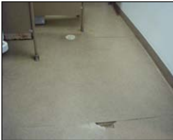
Floor Finishes: Replace Resilient Floor Finishes
