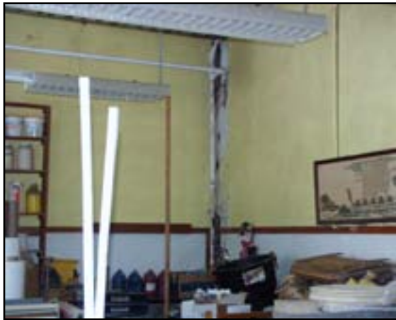
Partitions: Repair Water Damaged Walls
