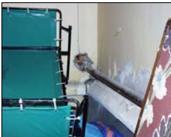
Substructure: Repair Below Grade Walls
