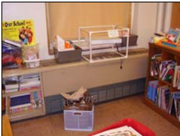
HVAC: Replace Classroom Unit Ventilators
