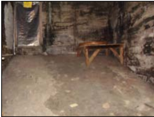
HVAC: Provide Negative Pressure in Crawlspace/Tunnels
