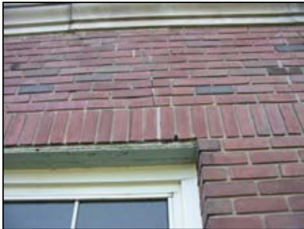
Exterior Walls: Grade-Level Wall Restoration
