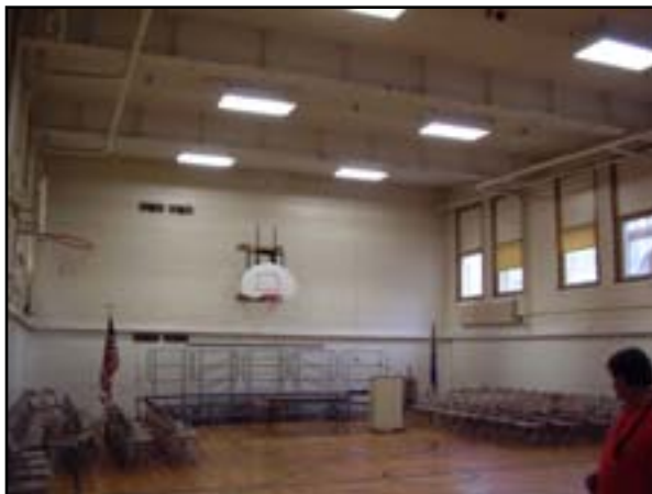
HVAC: Replace Ventilation in the Gym Auditorium/Cafeteria Areas
