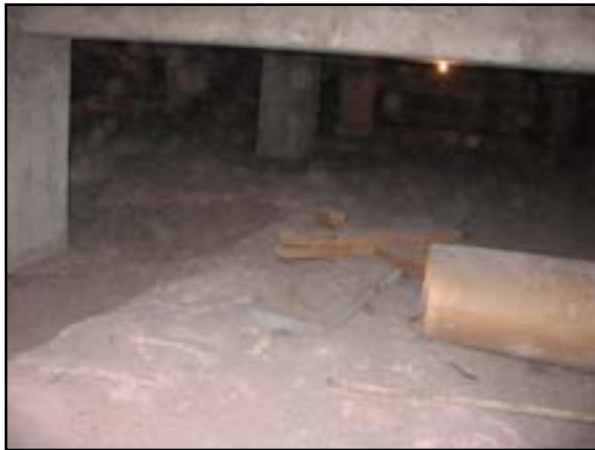
Service Tunnels: Floor Vapor Barrier
