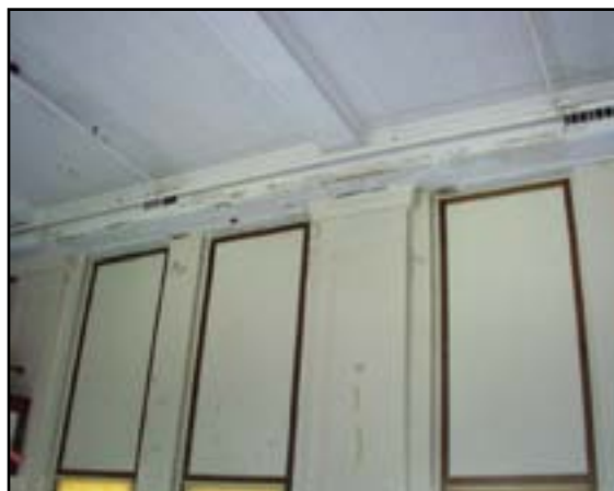
Wall Finishes: Repair Plaster
