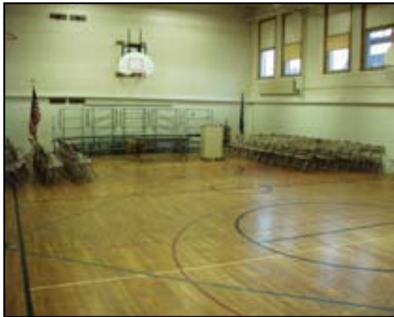
Floor Finishes: Refinish Gymnasium Floor
