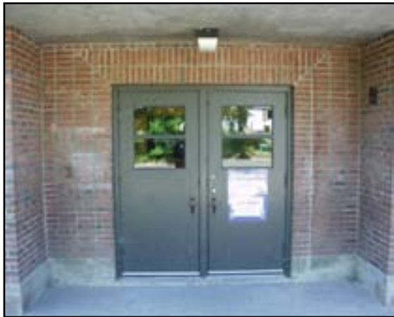
Exterior Doors: Replace Exterior Doors
