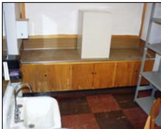
Equipment: Replace Cabinet Doors
