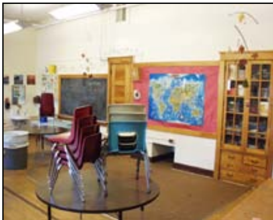
Floor Finishes: Refinish Wood Floors
