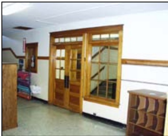
Interior Doors: Replace All Classroom Doors, Stairway Doors and Side Windows
