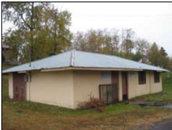
Exterior Walls: Wall Restoration
