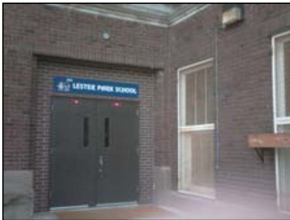
Communication and Security: Access Control
