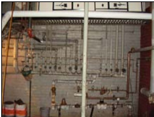
Plumbing: Replace Galvanized Domestic Water Piping
