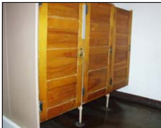
Fittings: Replace Toilet Partitions
