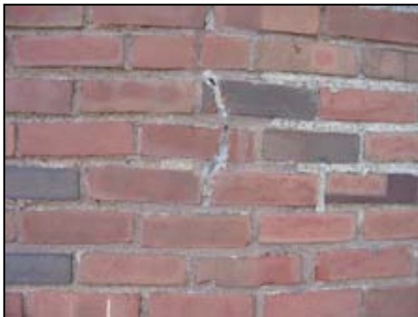
Exterior Walls: Roof-Level Wall Restoration
