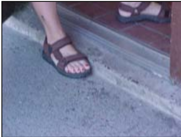
Site Improvements: Accessibility
