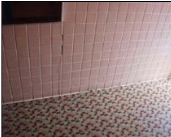
Wall Finishes: Replace Wall Tile in Boys and Girls Toilet Rooms
