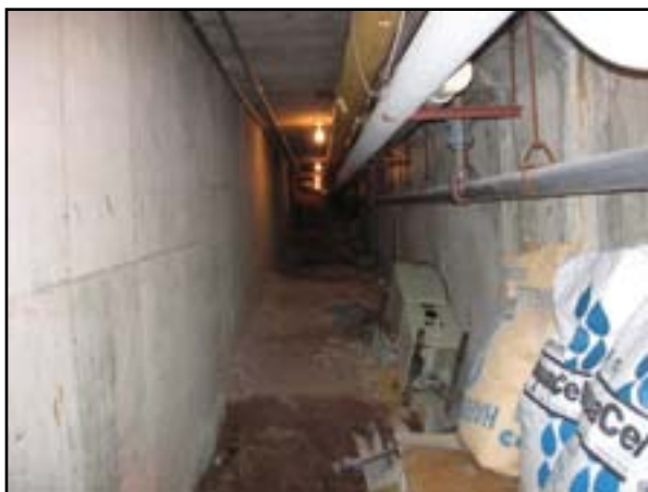
Service Tunnels: Floor Vapor Barrier
