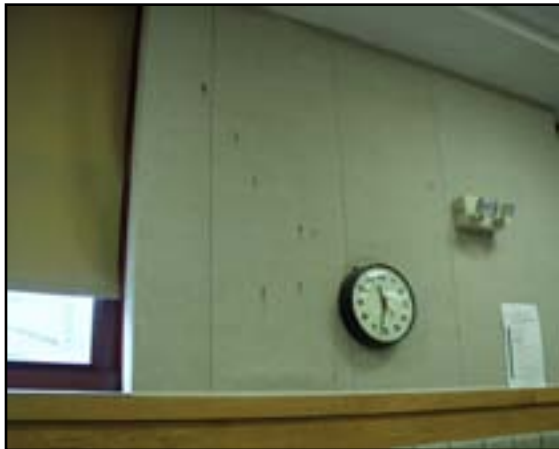
Wall Finishes: Replace Wall Panels at Cafeteria
