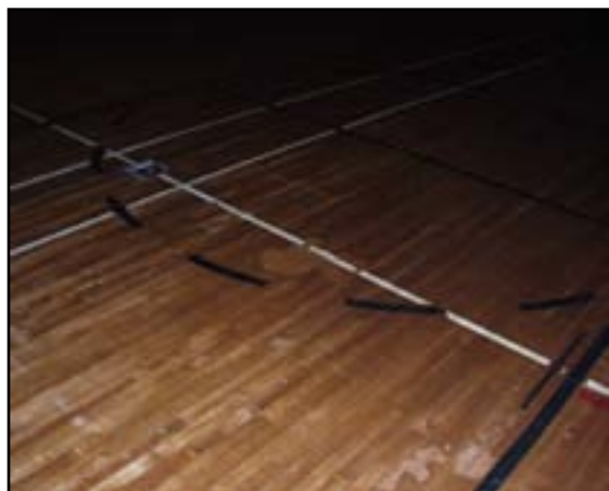
Floor Finishes: Refinish Gym Floor
