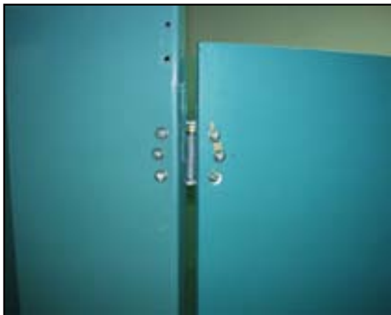
Fittings: Replace Toilet Partitions
