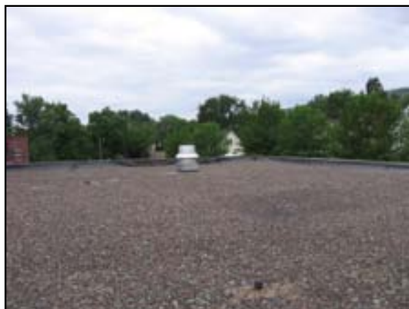
Roof System: Replace Roof
