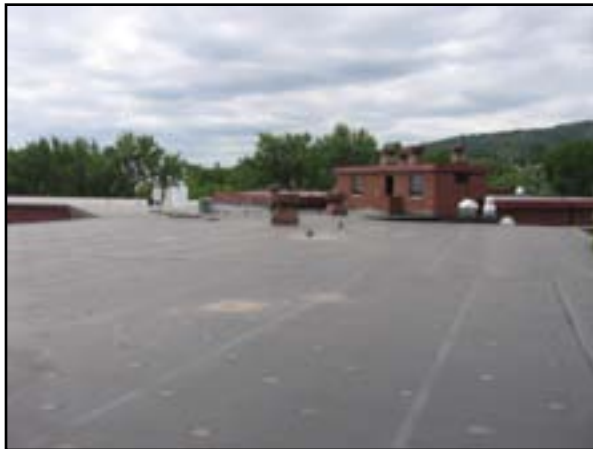
Roof System: Replace Roof
