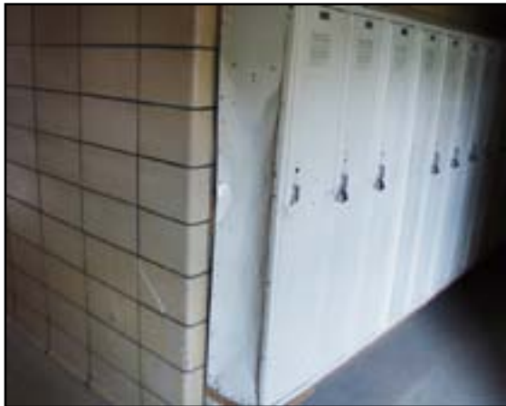
Equipment and Furnishings: Replace Damaged Student Lockers -
