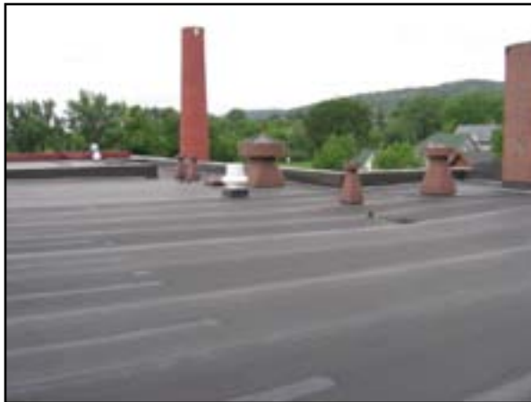
Roof System: Replace Roof
