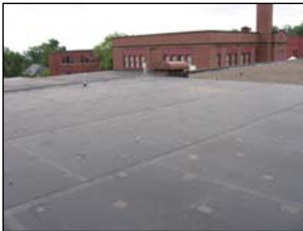
Roof System: Replace Roof
