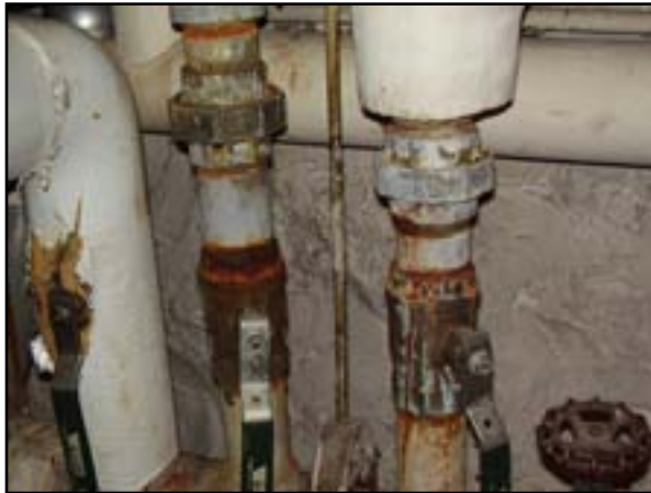
Plumbing: Replace Galvanized Domestic Water Piping
