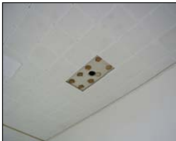
Ceiling Finishes: Install New Suspended Acoustical Ceiling
