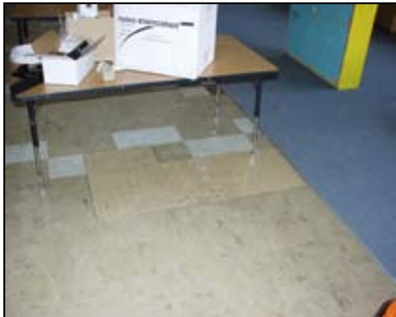
Floor Finishes: Replace VAT with VCT
