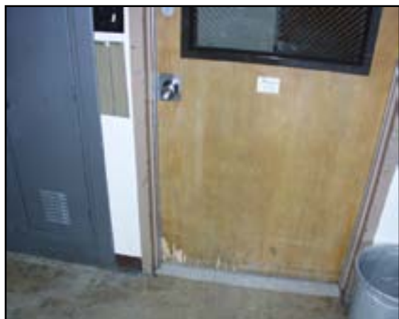
Interior Doors: Replace Classroom Corridor Doors
