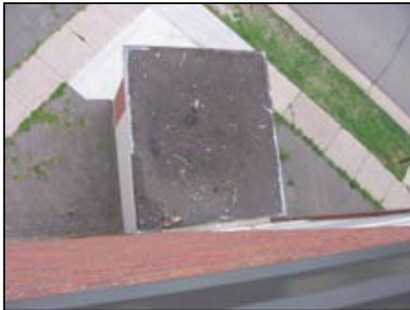
Roof System: Replace Roof
