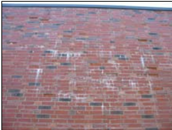
Exterior Walls: Wall Restoration
