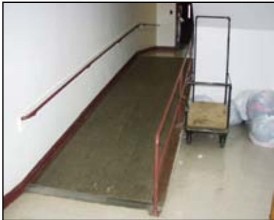
Superstructure: Reconstruct Ramp at 1889 Building
