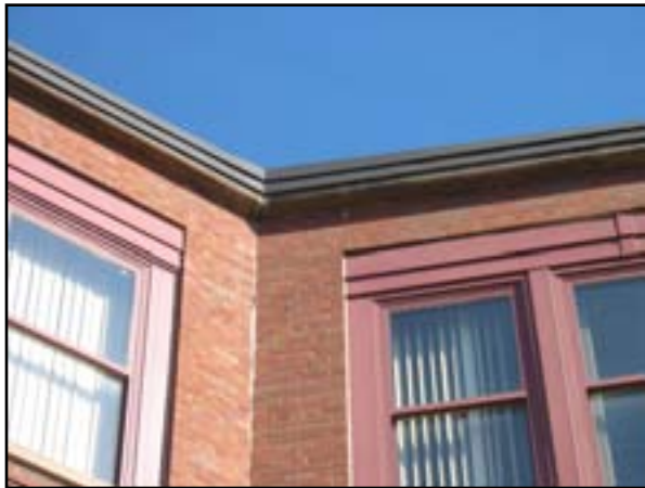
Exterior Walls: Wall Restoration
