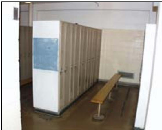
Superstructure: Refurbish Pool Locker Rooms
