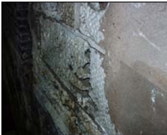
Substructure: Repair Leaking/Damaged Wall
