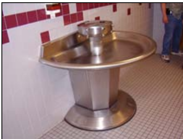
Plumbing: Replace Lavatory Wash Fountains
