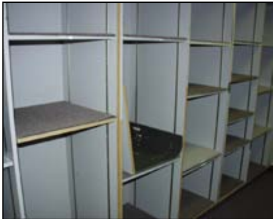
Equipment and Furnishings: Refurbish Casework
