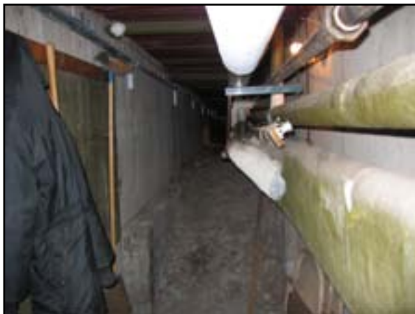
Service Tunnels: Floor Vapor Barrier
