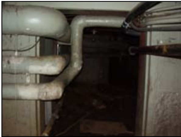
Plumbing: Relocate Sump Pump Discharge
