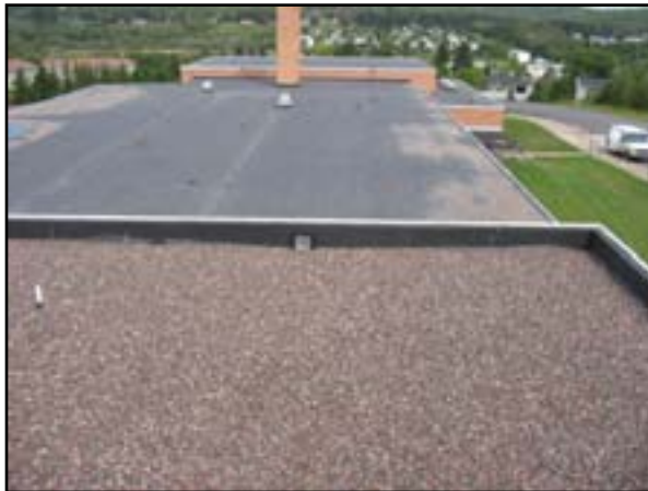
Roof System: Replace Roof
