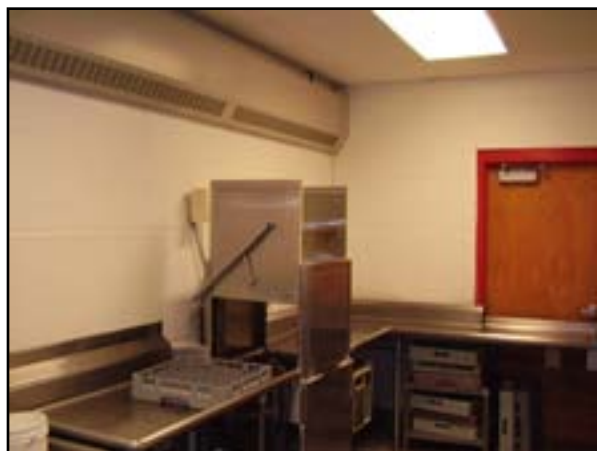
HVAC: Add Exhaust Hood to Dishwasher
