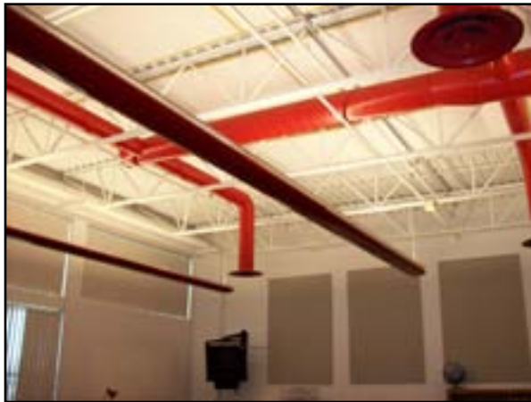
Wall Finishes: Paint Interior
