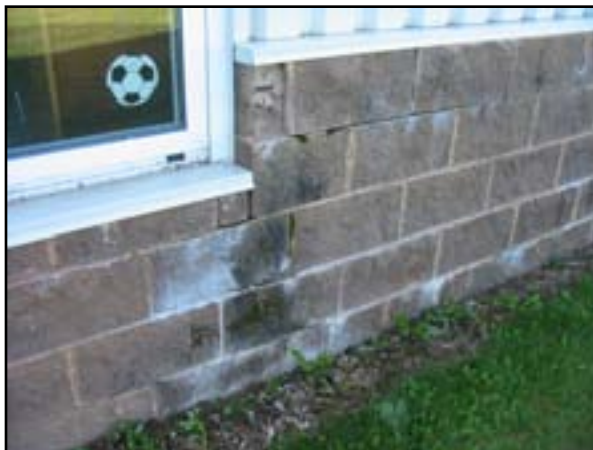
Exterior Walls: Wall Restoration
