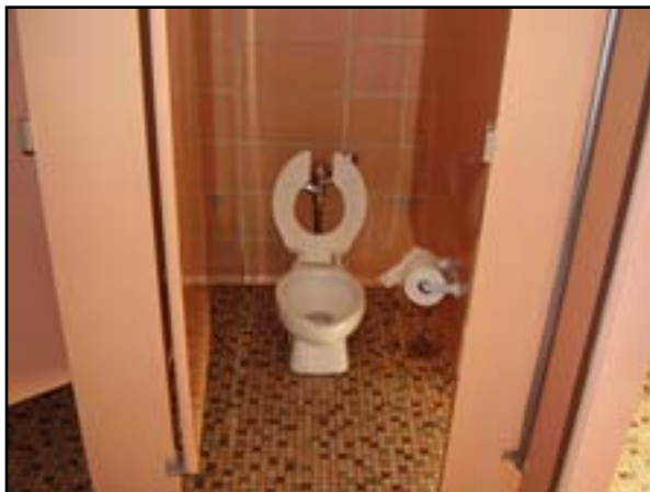
Plumbing: Replace Galvanized Domestic Water Piping
