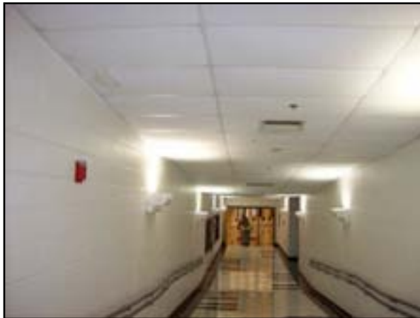
Ceiling Finishes: Acoustical Tile
