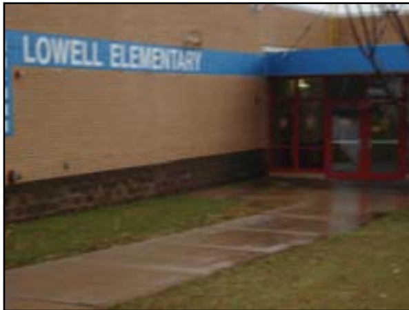
Communication and Security: Access Control
