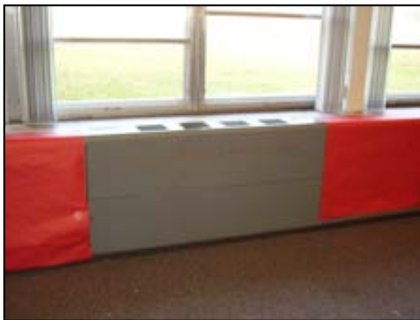
HVAC: Replace Classroom Unit Ventilators
