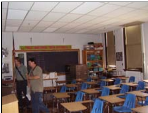
HVAC: Replace Ventilation All Floors 1916 Building Classrooms
