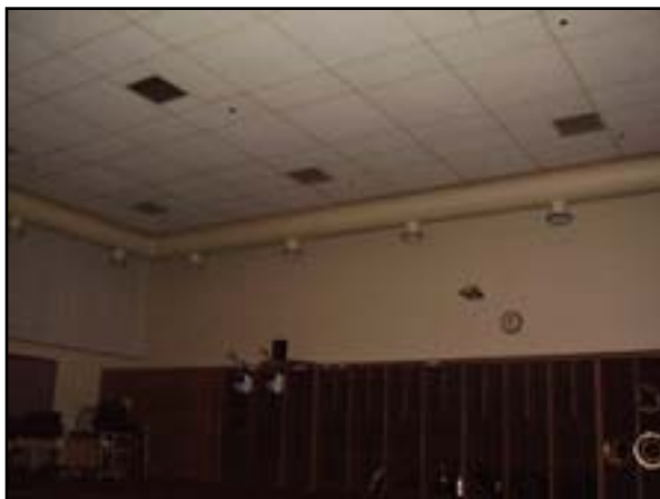
HVAC: Upgrade Ventilation and Add Dehumidification 1983 Music Addition
