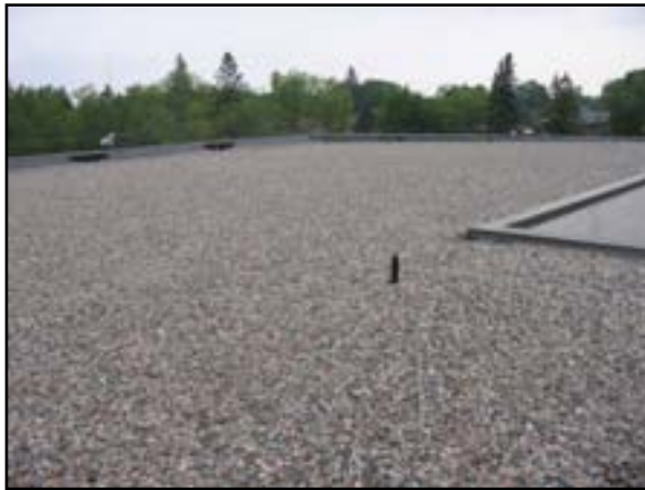
Roof System: Replace Roof
