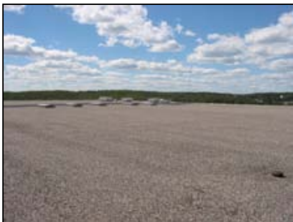
Roof System: Replace Roof
