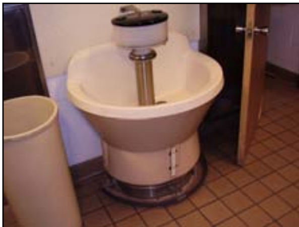
Plumbing: Replace Lavatory Wash Fountains
