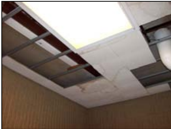
Ceiling Finishes: Replace Suspended Acoustical Tile
