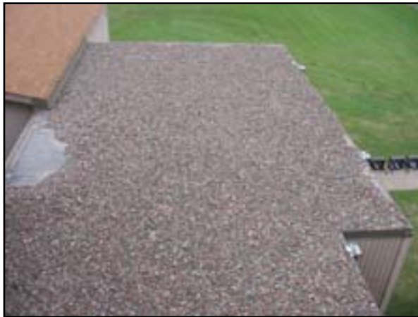
Roof System: Replace Roof
