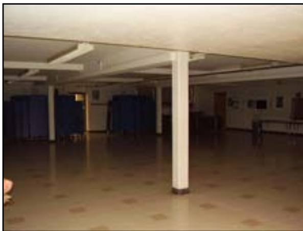
HVAC: Replace Ventilation in the Gym/Auditorium/Cafeteria Areas
