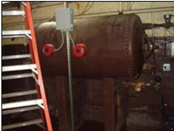
Plumbing: Replace Domestic Water Heat Exchanger
