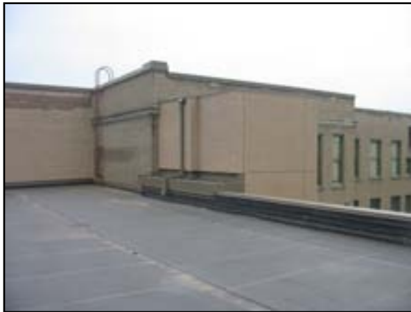
Exterior Walls: Roof-Level Wall Restoration
