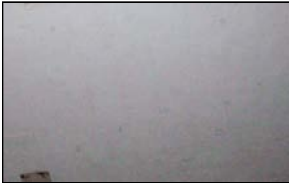
Ceiling Finishes: Replace Ceiling with Sanitary, Washable Tile
