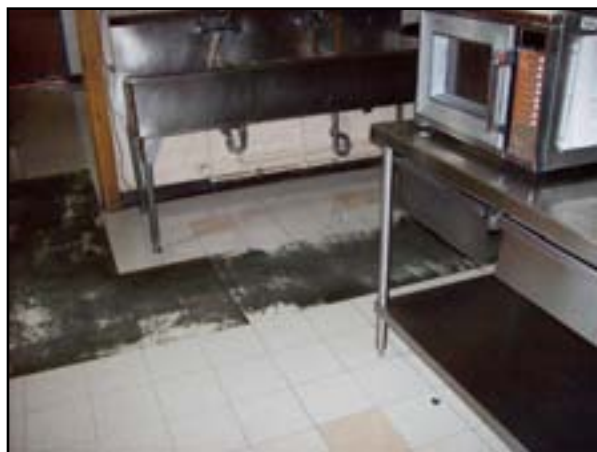
Floor Finishes: Replace Vinyl Tile
