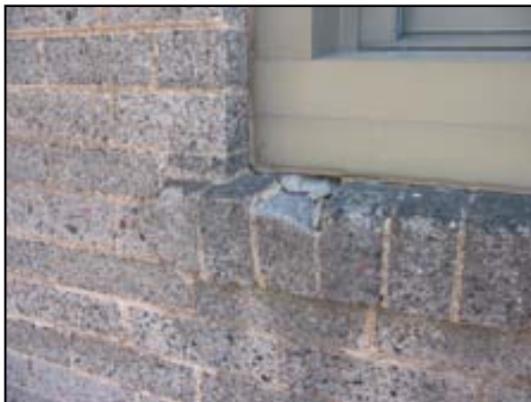
Exterior Walls: Wall Restoration
