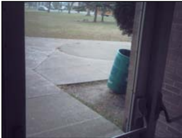
Communication and Security: Access Control
