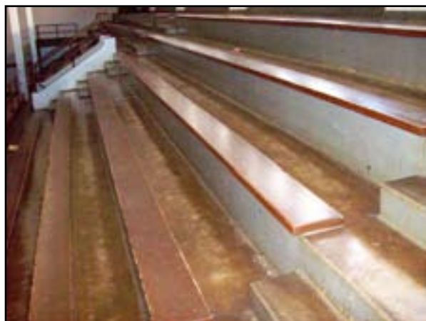
Equipment and Furnishings: Refinish Balcony Seats
