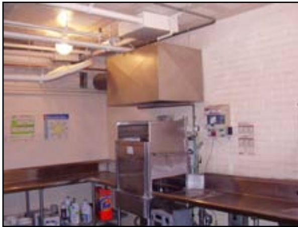
HVAC: Replace Dishwasher Exhaust Hood
