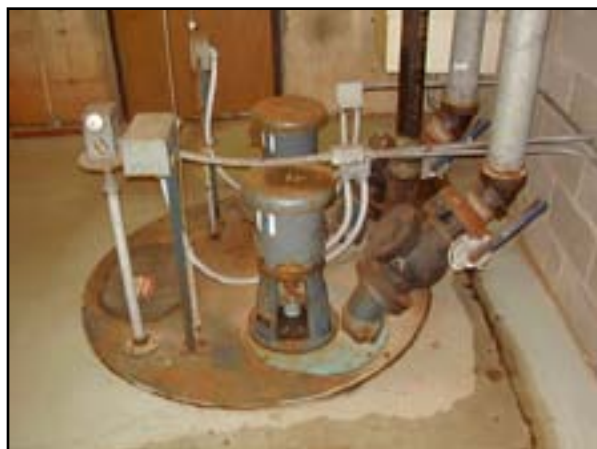
Plumbing - Sump Pump Replacement
