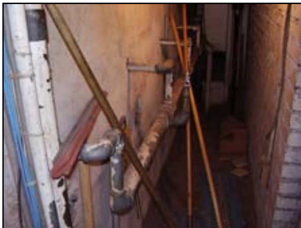
Plumbing: Replace Galvanized Domestic Water Piping
