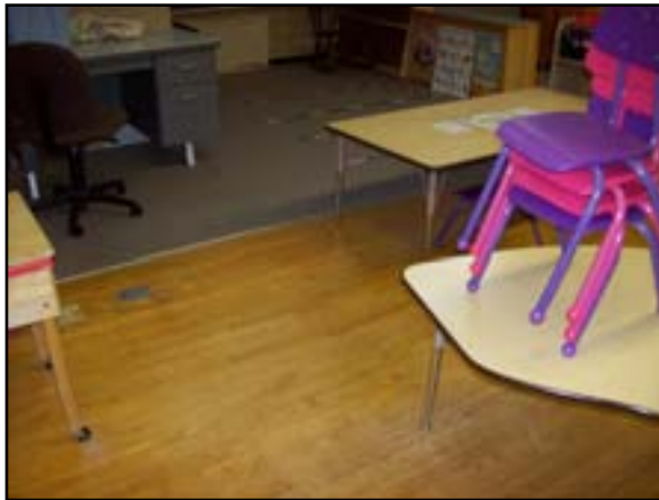
Floor Finishes: Refinish Hardwood Floors
