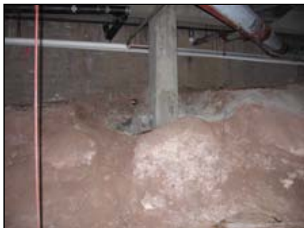
Service Tunnels: Floor Vapor Barrier
