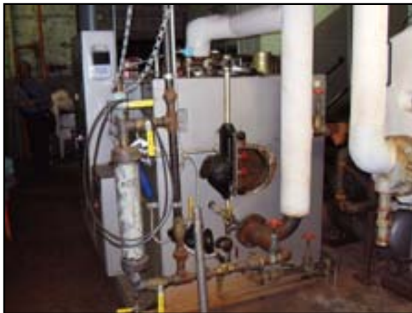
HVAC: Heating System Conversion - Steam to Hot Water
