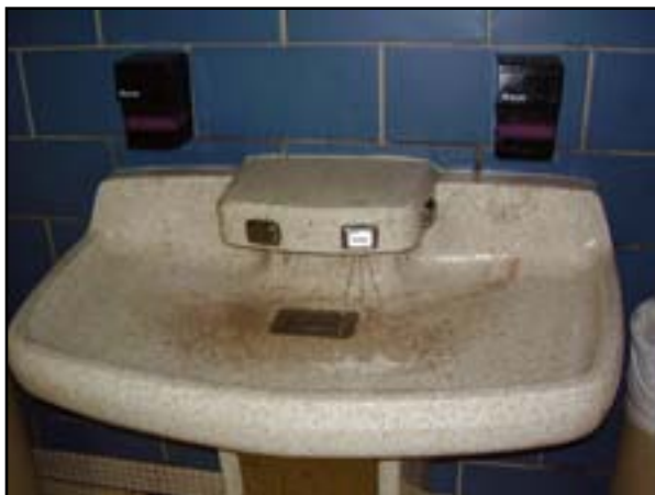
Plumbing: Replace Lavatory Wash Fountains
