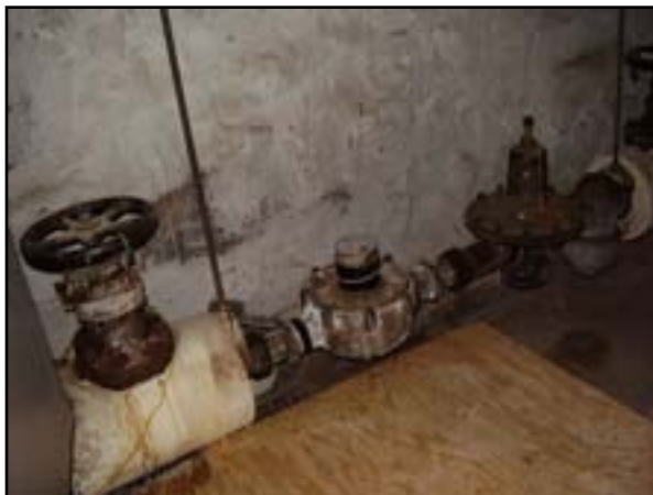
Plumbing: Replace Galvanized Domestic Water Piping
