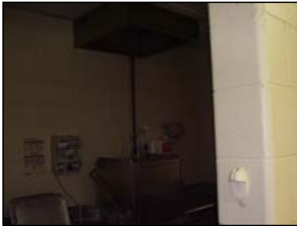
HVAC: Replace Dishwasher Exhaust Hood
