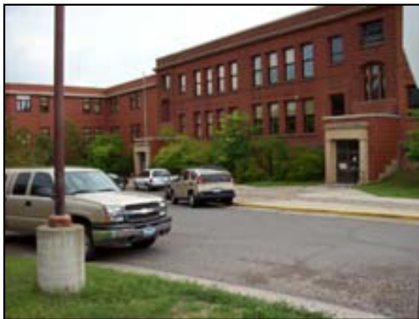
Exterior Windows: Replace Windows
