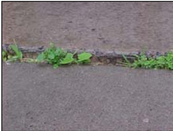
Site Improvements: Accessibility
