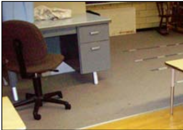
Floor Finishes: Replace Carpet
