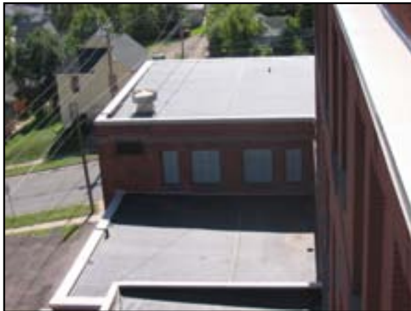
Roof System: Replace Roof
