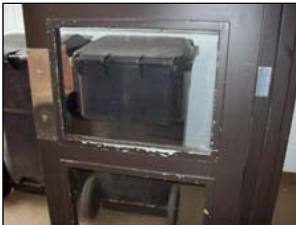
Exterior Doors: Paint Doors
