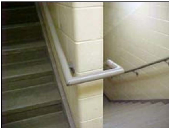
Interior Construction: Accessibility
