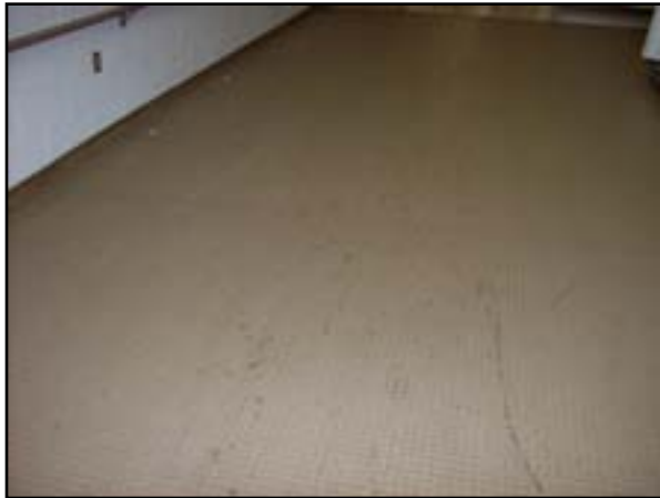
Floor Finishes: Replace Rubber Flooring
