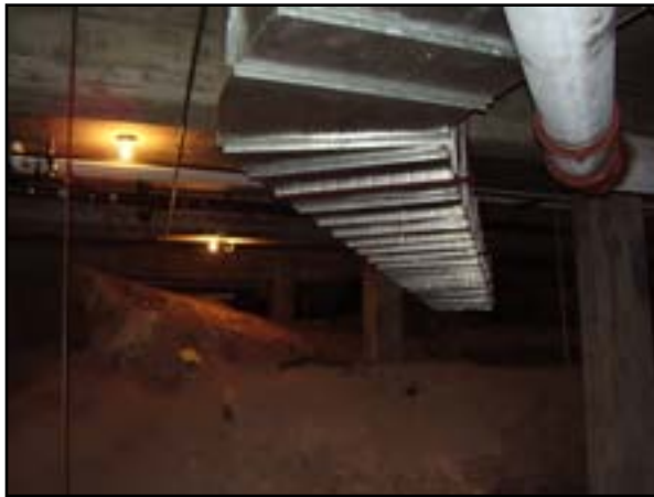
HVAC: Provide Negative Pressure in Crawlspace/Tunnels
