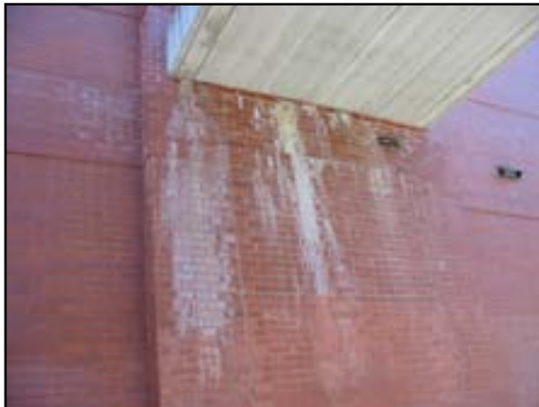
Exterior Walls: Grade-Level Wall Restoration
