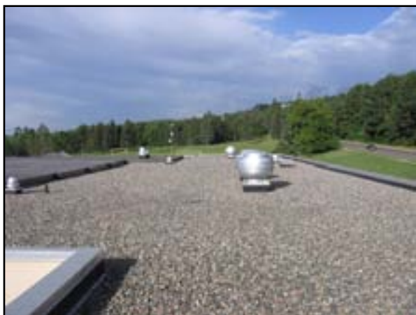
Roof System: Replace Roof
