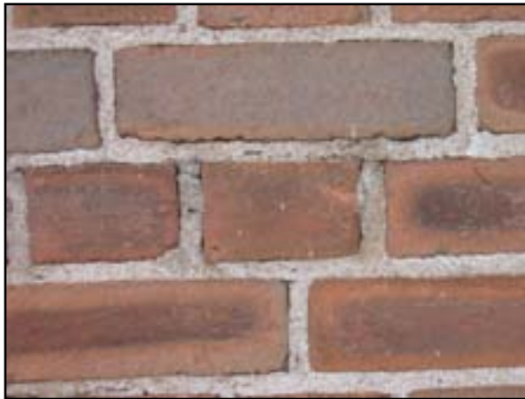
Exterior Walls: Wall Restoration
