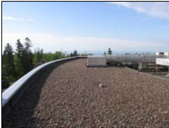
Roof System: Replace Roof
