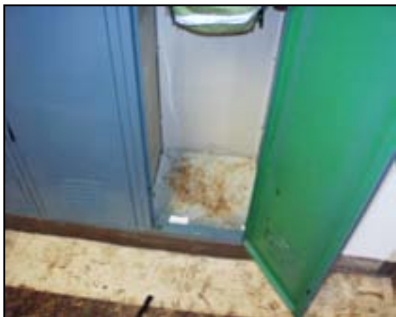
Fittings: Replace Existing Lockers
