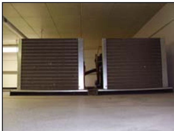
HVAC: Remote Condenser Heat Removal
