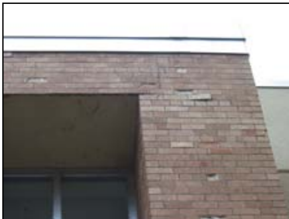
Exterior Walls: Grade-Level Wall Restoration
