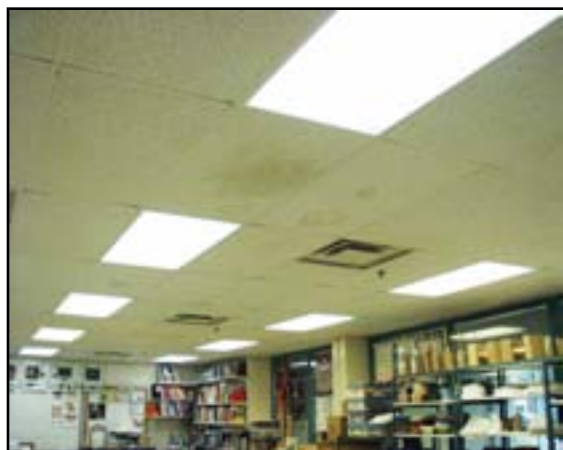
Ceiling Finishes: Replace 2x4 Acoustical Tile
