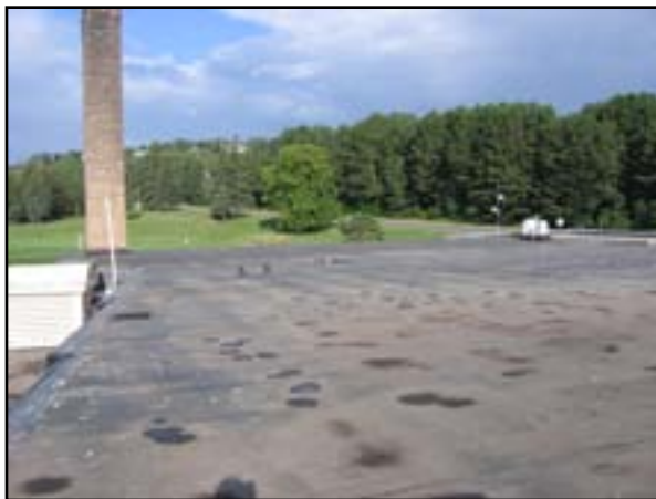
Roof System: Replace Roof
