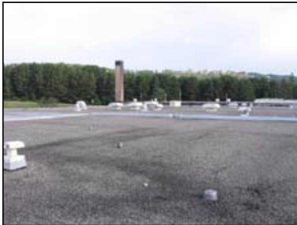
Roof System: Replace Roof
