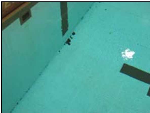
Aquatic Facilities: Pool inlets and grout
