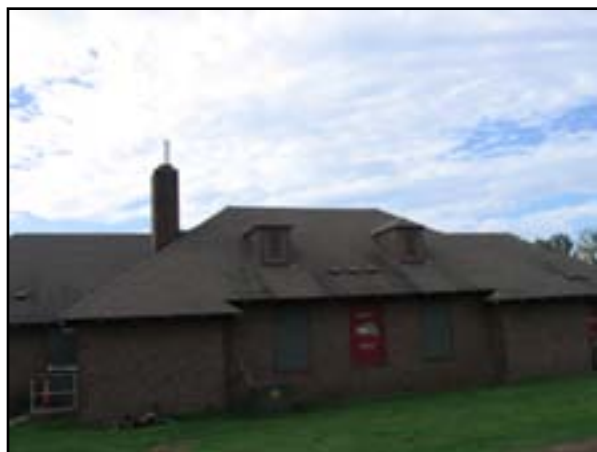
Roof System: Replace Roof
