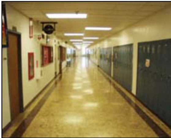
Wall Finishes: Interior Paint
