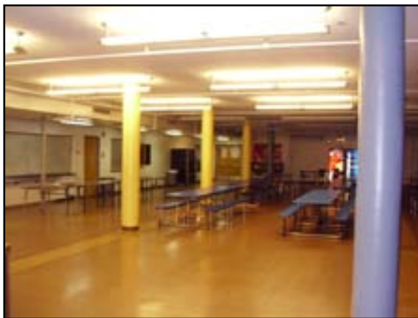
HVAC: Replace Ventilation in the Gym/Auditorium/Cafeteria Areas
