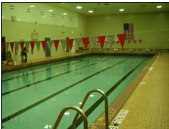
HVAC: Pool Unit Replacement along with an Automatic Pool Cover
