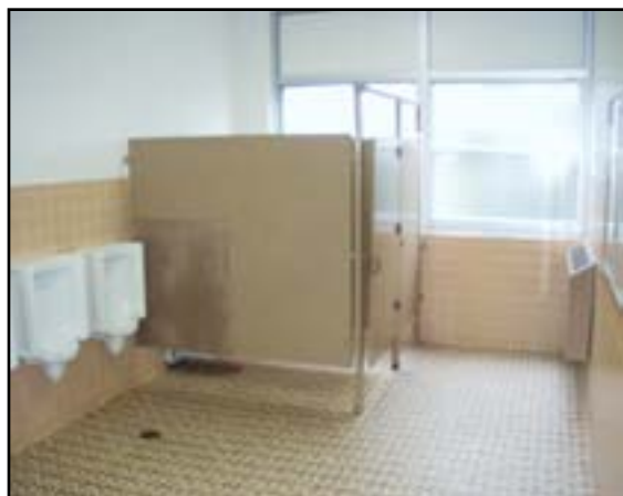
Fittings: Replace Toilet Partitions
