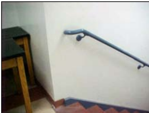
Interior Construction: Accessibility
