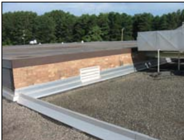
Exterior Walls: Roof-Level Wall Restoration
