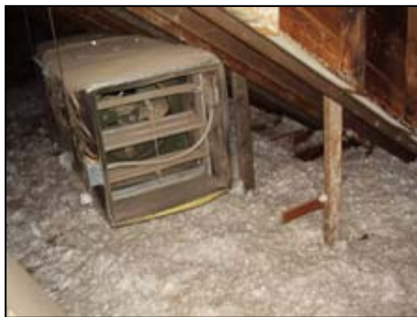
HVAC: Add Relief Ductwork and Louvers/Hoods
