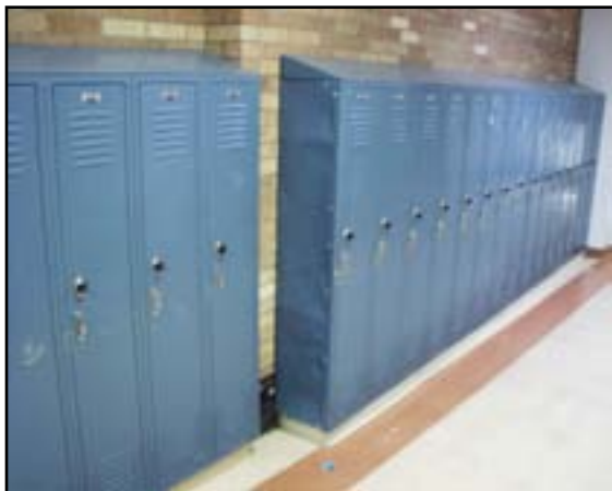
Fittings: Replace Existing Lockers
