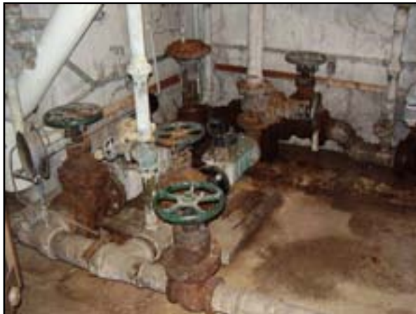
Plumbing: Replace Galvanized Domestic Water Piping
