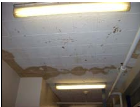
Ceiling Finishes: Replace 12x12 Acoustical Tile
