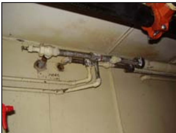
Plumbing: Replace Galvanized Domestic Water Piping
