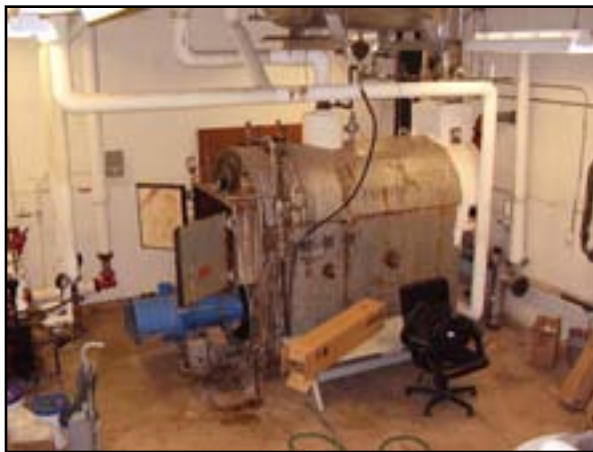
HVAC: Boiler Room Upgrades
