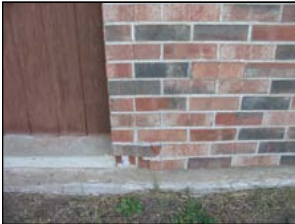
Exterior Walls: Wall Restoration
