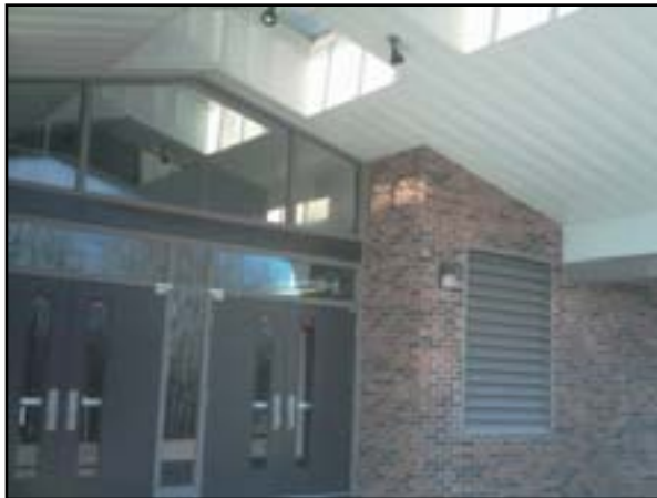
Communication and Security: Access Control -
