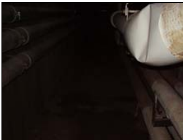
HVAC: Provide Negative Pressure in Crawlspace/Tunnels
