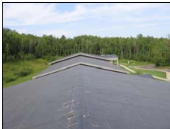
Roof System: Replace Roof
