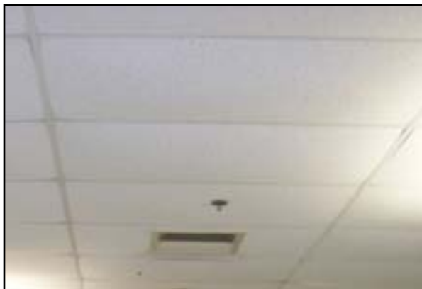
Ceiling Finishes: Replace Acoustical Tile
