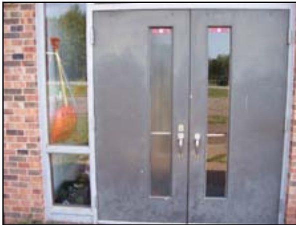
Exterior Doors: Paint Doors
