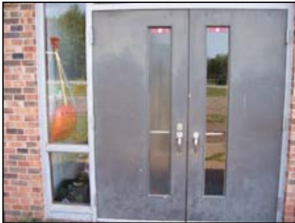
Exterior Doors: Paint Doors
