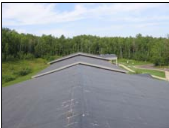
Roof System: Replace Roof
