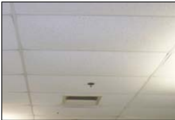
Ceiling Finishes: Replace Acoustical Tile
