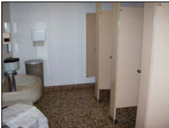
Superstructure: Reconstruct Toilet Rooms for Accessibility
