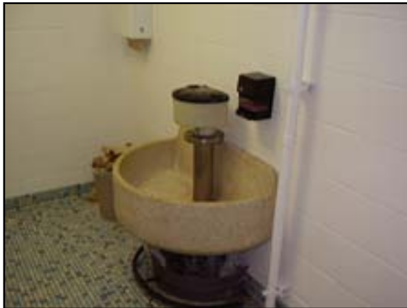
Plumbing: Replace Lavatory Wash Fountains
