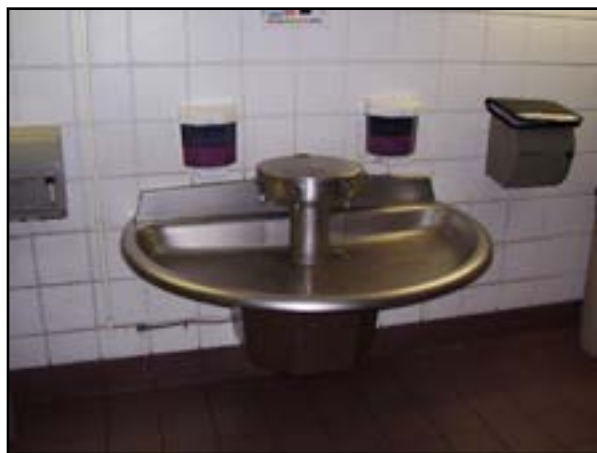
Plumbing: Replace Lavatory Wash Fountains
