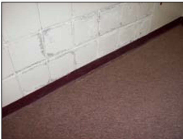
Wall Finishes: Paint Interior
