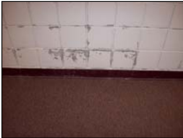
Wall Finishes: Repair Water Damage
