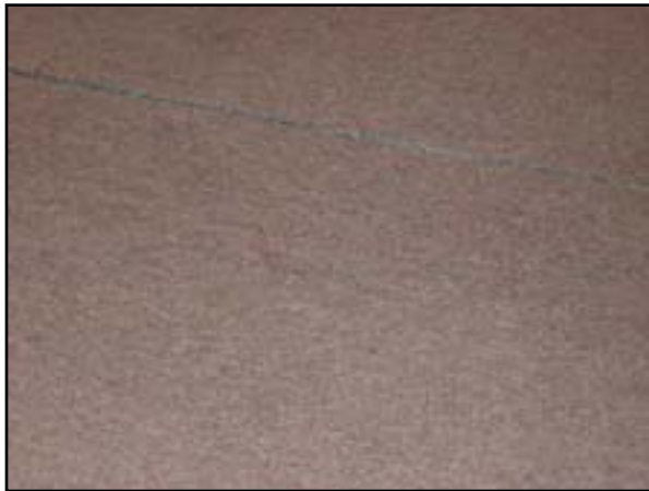
Floor Finishes: Replace Corridor Carpet -
