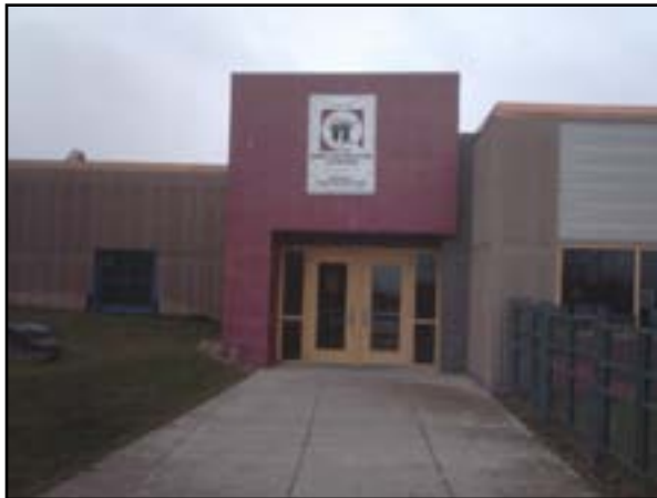
Communication and Security: Access Control
