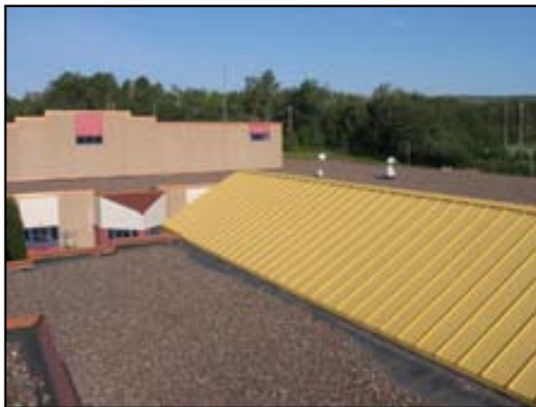
Roof System: Replace Roof
