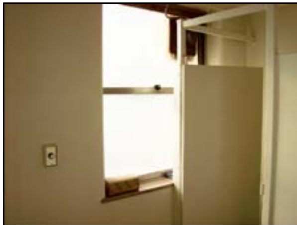
Exterior Windows: Steel Windows
