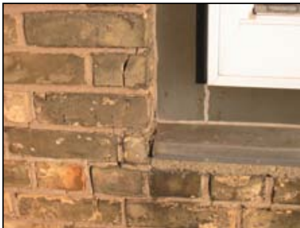
Exterior Walls: Wall Restoration
