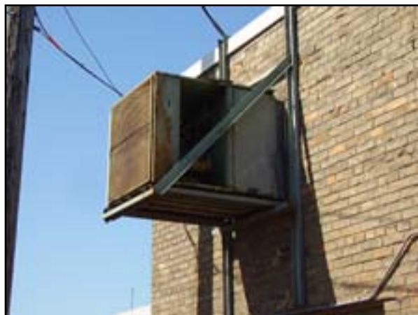
HVAC: Upgrade Office Ventilation and Add Dehumidification
