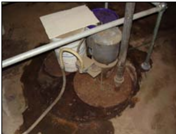
Plumbing - Sump Pump Replacement
