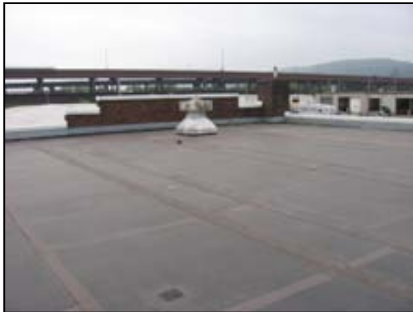
Roof System: Replace Roof
