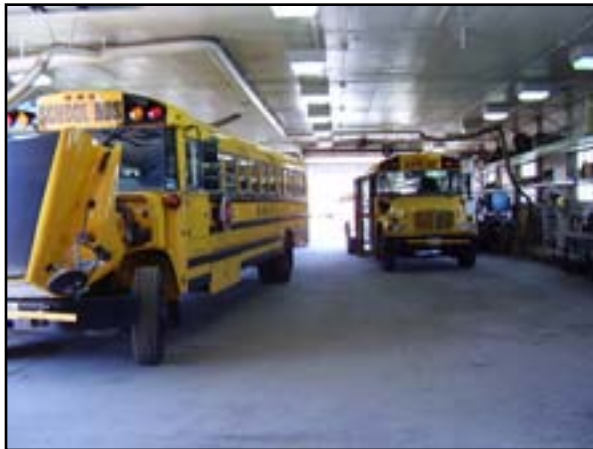
HVAC: Ventilation Improvements - Shop
