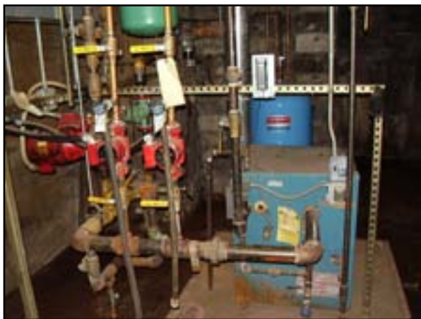
HVAC: Boiler Room Upgrades
