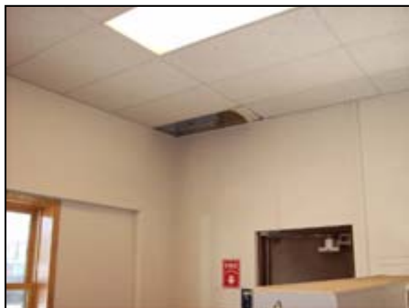
Ceiling Finishes: Suspend Acoustical Tile
