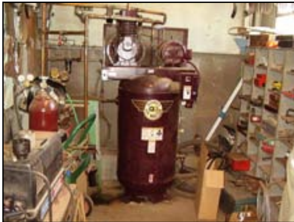
Plumbing: Upsize Service Air Lines
