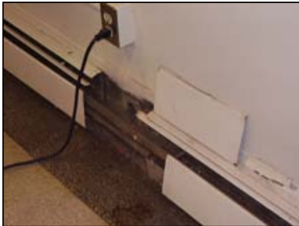
HVAC: Add Propylene Glycol to Heating System
