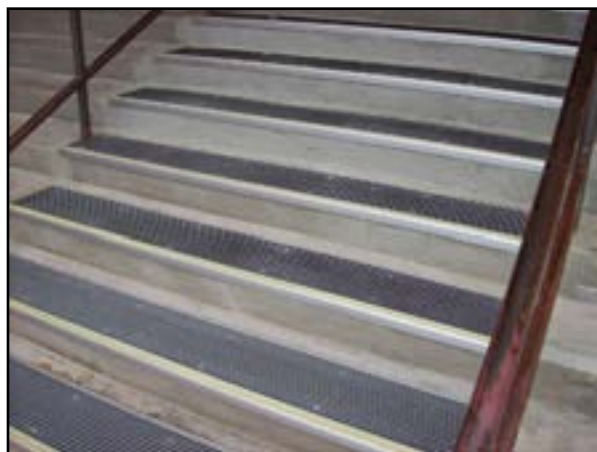
Stairs: Replace Applied Non-slip Treads
