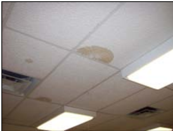
Ceiling Finishes: Replace Acoustical Tile
