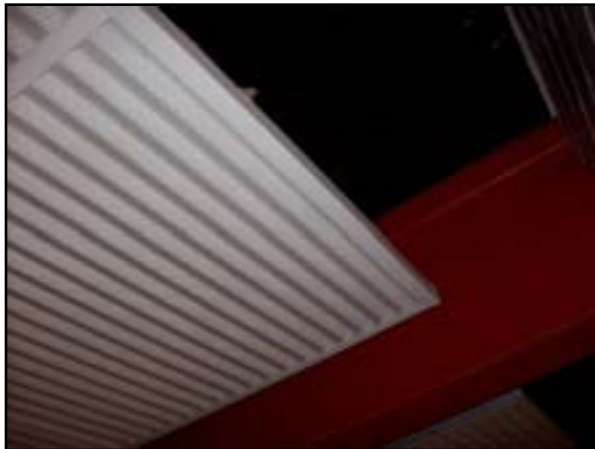
Ceiling Finishes: Replace Perforated Acoustical Metal Panels
