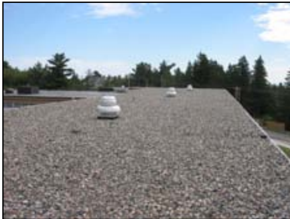
Roof System: Replace Roof
