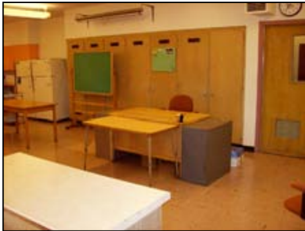
Fittings: Replace Chalkboard
