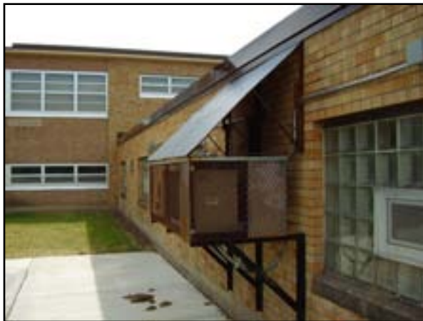
Kitchen Equipment: Replace Remote Kitchen Condensers
