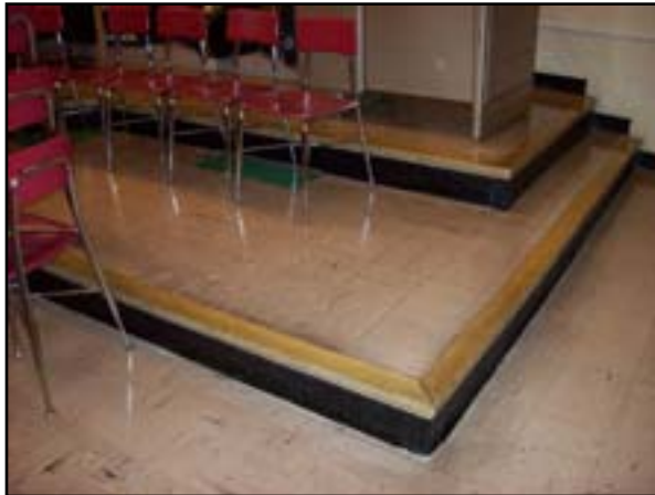
Floor Finishes: Replace VAT
