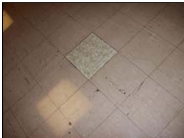
Floor Finishes: Replace Kitchen Flooring
