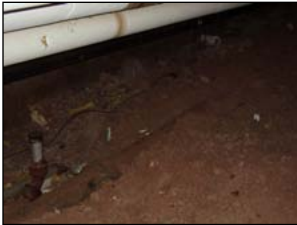
Plumbing: Replace Underground Sanitary Sewer Mains in Crawlspace/Tunnel Areas
