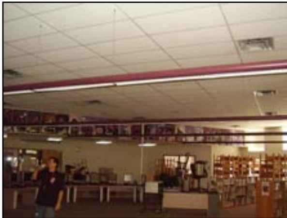
HVAC: Add Dehumidification 1994 Units
