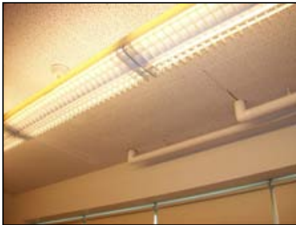
Ceiling Finishes: Replace Acoustical Tile
