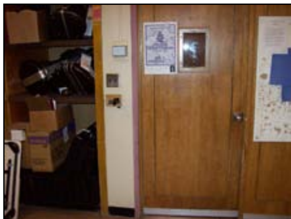
Interior Doors: Refinish Wood Doors
