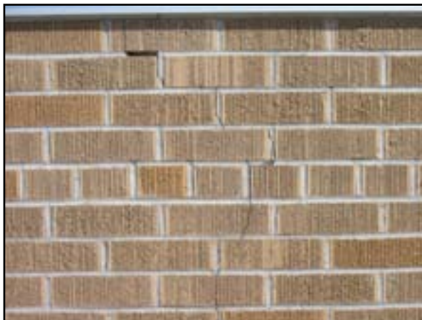
Exterior Walls: Wall Restoration
