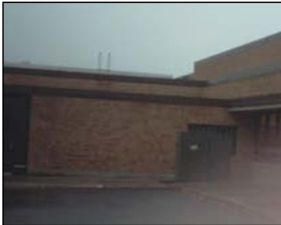
Emergency Power Distribution: Generator Backup
