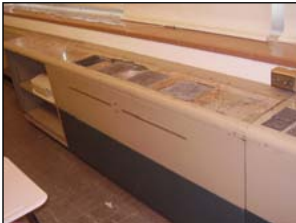
HVAC: Replace Classroom Unit Ventilators
