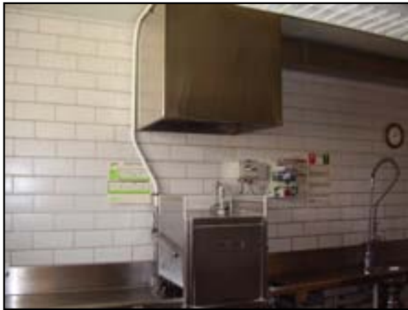
HVAC: Replace Dishwasher Exhaust Hood
