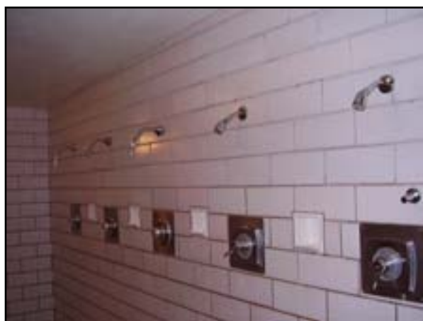
Plumbing: Replace Galvanized Domestic Water Piping
